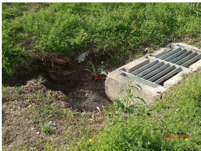
Figure 26: Erosion around Drop Inlet East of Paige Road.
