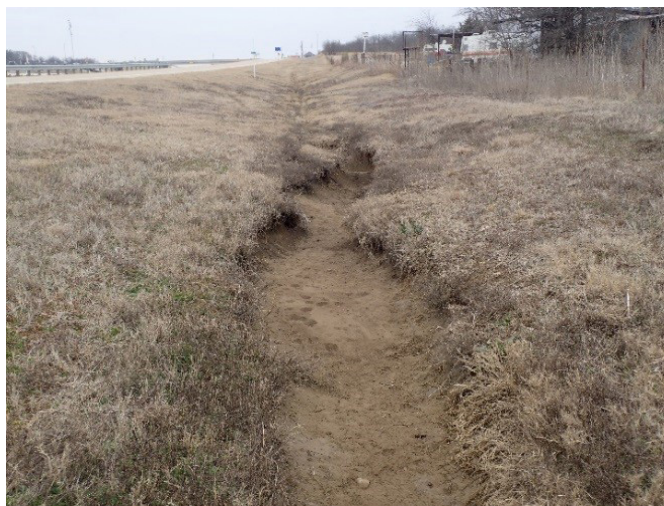
Figure 31: Ditchline Erosion NB Exit Ramp to FM 917
