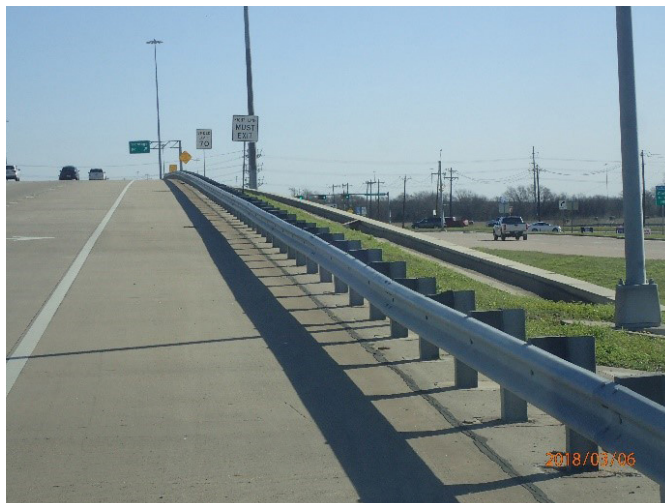
Figure 27: Missing Delineation at NBML West of Hardin Blvd.
