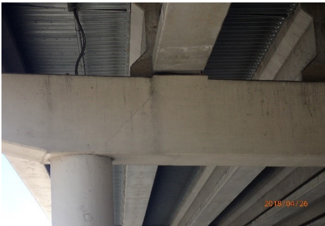
Figure 15: Cap Cracking EB Center Bent to Coit Road.
