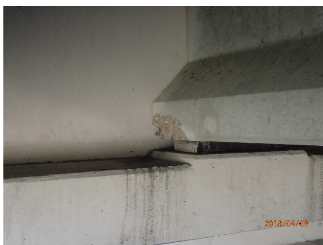
Figure 29: Beam end spalling at SBML @ Huffines Blvd. bridge.
