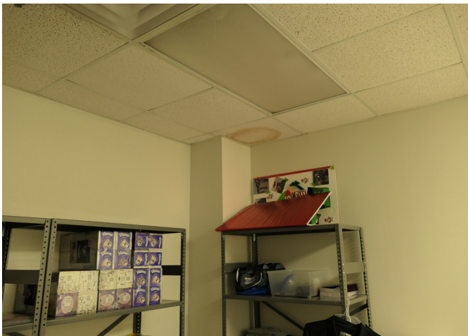
Figure 19: MLP7 Evidence of water intrusion.
