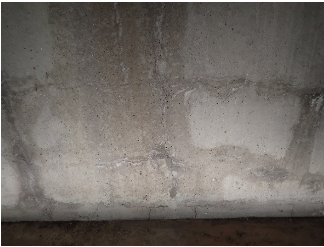
Figure 33: Bridge Backwall Cracking at Sparks Drive.
