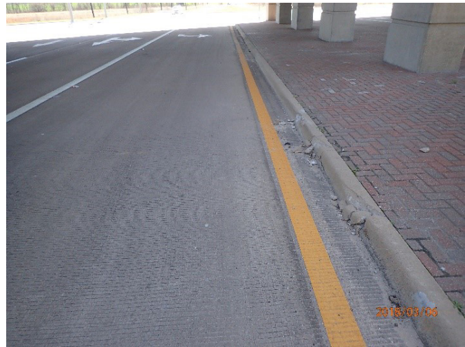
Figure 24: Broken curb at Hardin Blvd.
