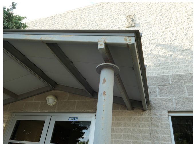
Figure 37: Rust on West Entry Canopy at Gleneagles Office Center.
