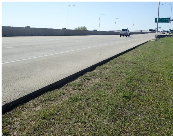
Figure 30: Example of Pavement Edge Drop Off at various locations.
