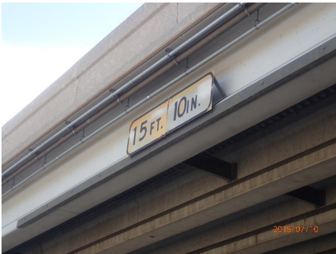
Figure 4: Clearance Sign Faded at EB Briargrove.
