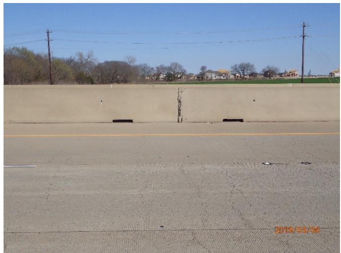
Figure 25: Barrier Spall NB West of Lake Forest Drive.
