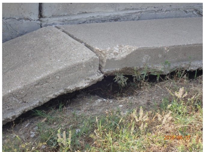
Figure 2: Erosion at Mow Strip SB DNT at Cotton Gin Road.
