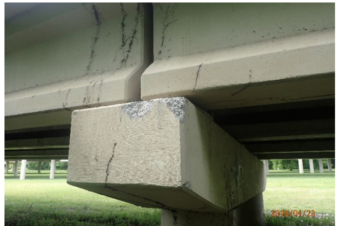
Figure 18: Cap Damage WB Exit Ramp to Brand Road.
