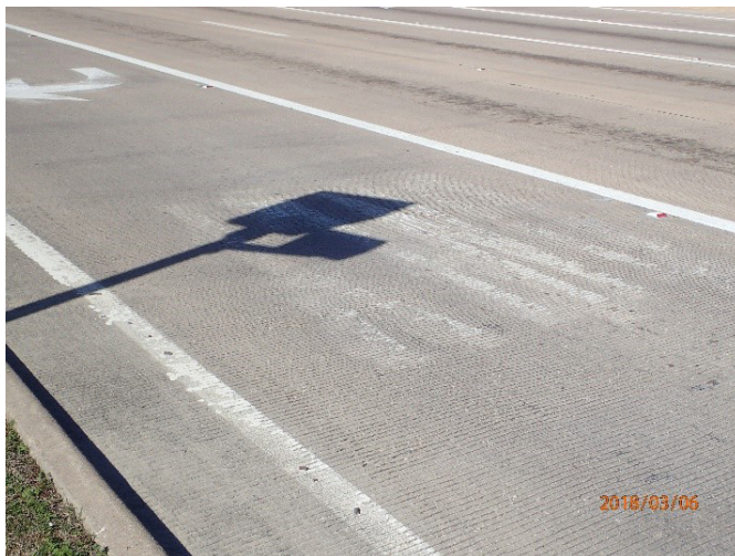
Figure 22: Faded Striping and Graphics NBFR West of Custer Road.
