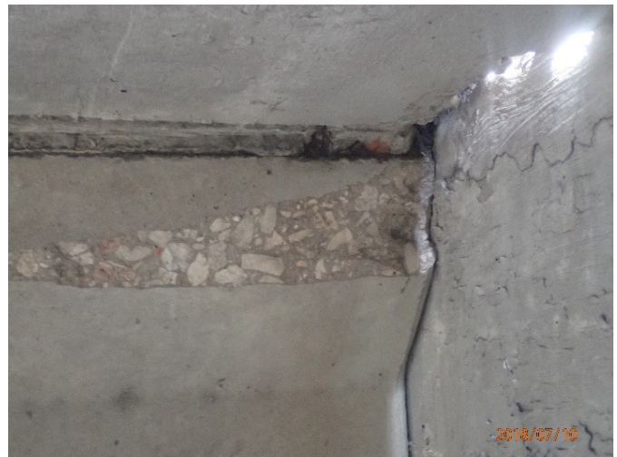
Figure 8: Beam end spalling SB DNT at Spring Valley.
