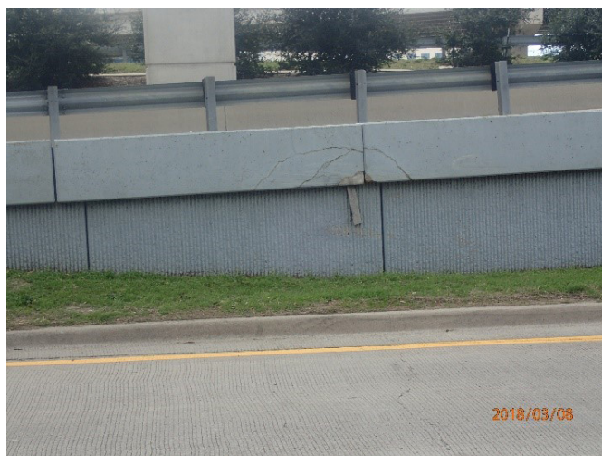
Figure 28: Minor Coping Damage SBFR East of Dallas North Tollway.
