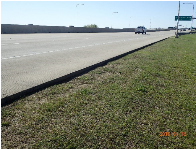
Figure 12: Pavement Edge Drop Off North of Merritt Road.
