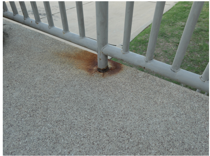
Figure 36: Rust Damage to Pipe at Ohio Drive Maintenance Service Center.
