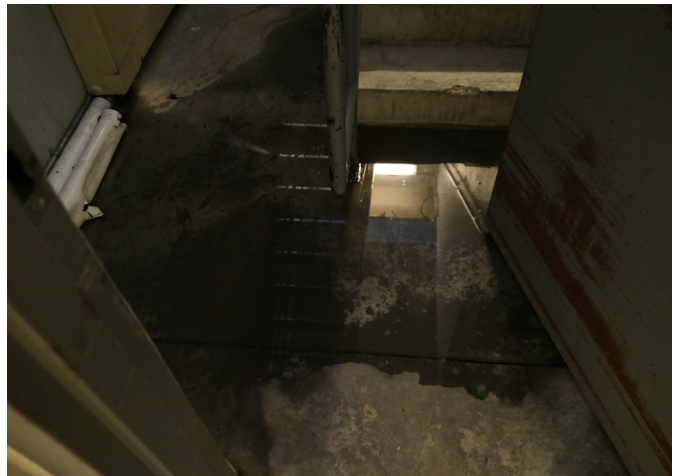
Figure 20: MLP7 Standing Water at Booth Access Stairs.
