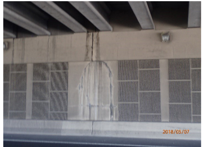
Figure 13: Retaining Wall Cracking EB PGBT under Old Denton Road.
