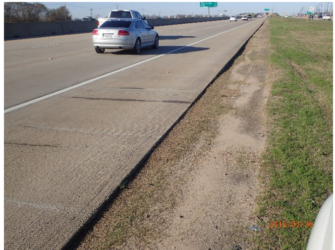
Figure 23: Pavement Edge Drop-off SBML at County Road 149.
