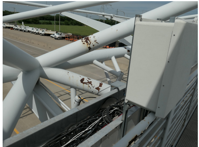
Figure 10: MLP 4 Rust on exterior railings
