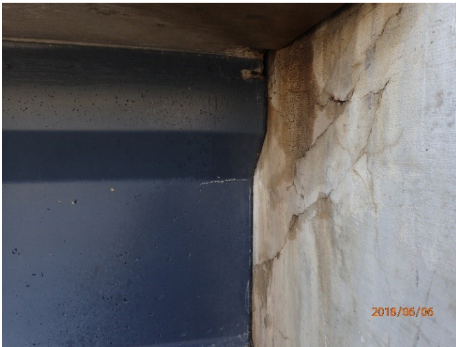
Figure 9: Backwall Cracking SB DNT at Rock Hill.
