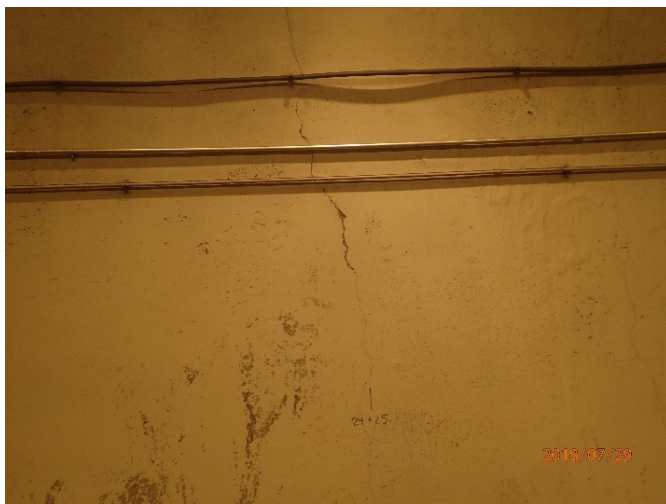
Figure 35: Cracking on tunnel wall.
