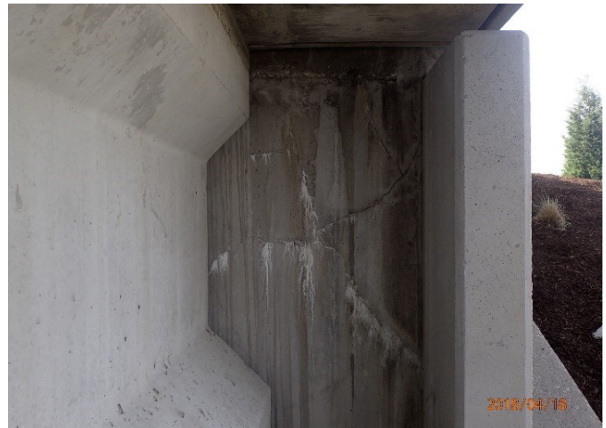
Figure 17: Cracks with Efflorescence SBML North of Valley View Lane.
