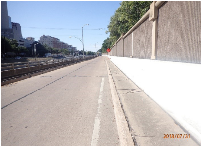
Figure 3: Faded Striping at SB Entrance Ramp from Northwest Highway.
