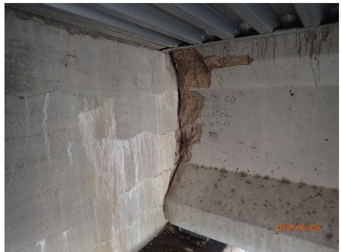
Figure 7: Beam end spalling and backwall cracking NB DNT at Rock Hill South Abutment.
