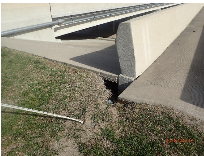
Figure 16: Erosion & Undermining of Riprap at Merritt Road.
