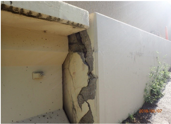
Figure 14: Backwall Cracking & Spalling EB Relief Bridge between Preston and DNT.
