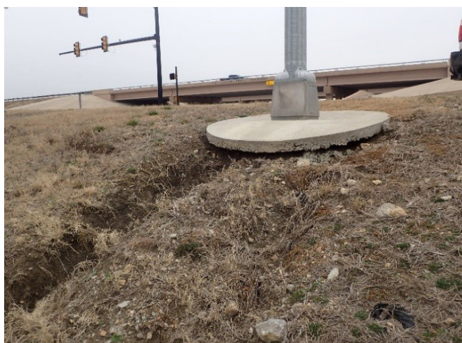
Figure 32: Erosion Around Luminaire Riprap SB Ramp from Sycamore School Road
