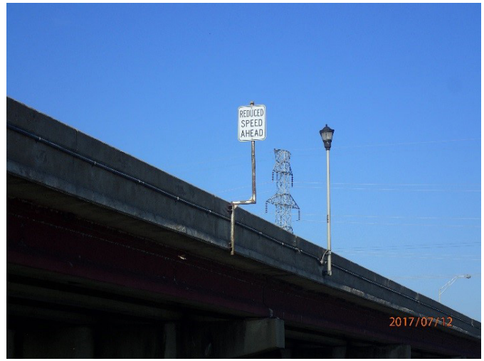
Figure 34: Rusty sign posts on bridge.
