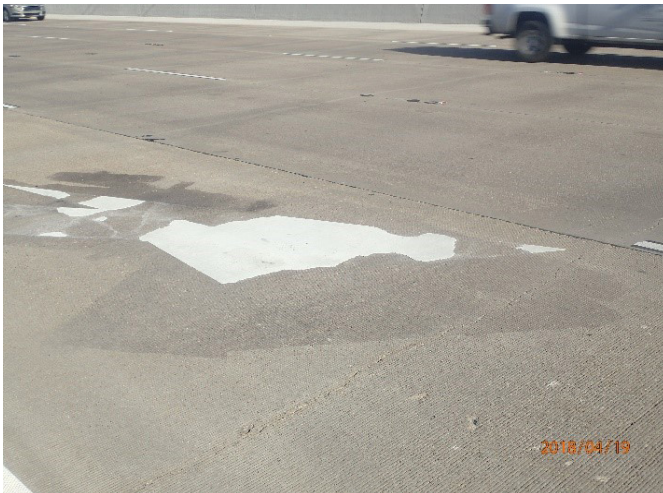
Figure 11: Striping Cracked & Missing (arrow) EB PGBT E of Water View.
