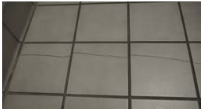
Figure 51: Gleneagles 5900 crack in floor tile
