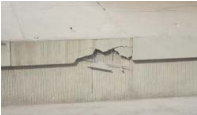
Figure 33: SRT coping damage NBML at Castle Hills
