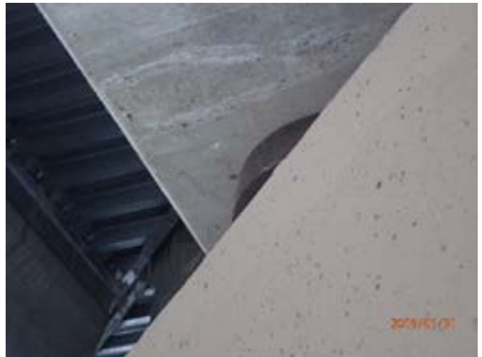
Figure 42: CTP bearing pad movement
