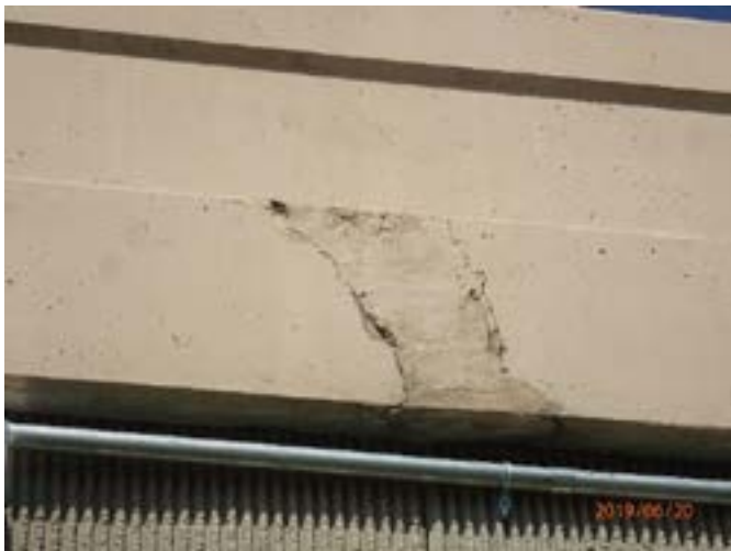
Figure 8: DNT coping damage NB north of Harvest Hill Road
