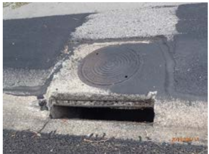
Figure 7: DNT curb inlet damage with steel exposed NB south of Lovers Lane
