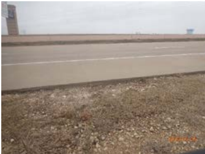
Figure 37: CTP pavement edge drop off
