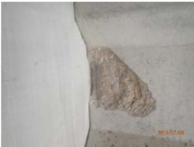
Figure 10: DNT beam spall SB at Panther Creek
