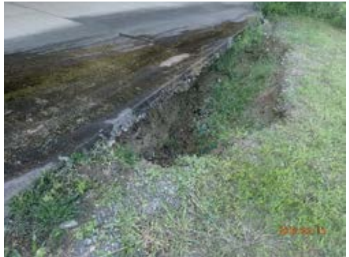
Figure 22: PGBT erosion at bridge riprap WB at Royal Lane
