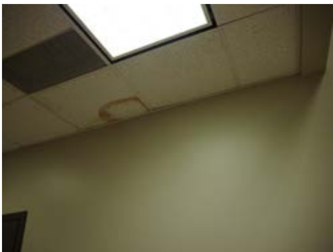
Figure 12: DNT MLP3 – staining on ceiling tile
