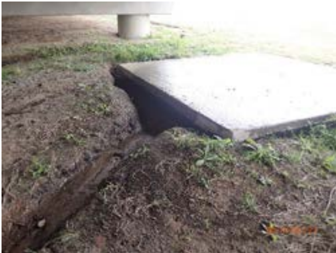
Figure 39: CTP erosion at structure
