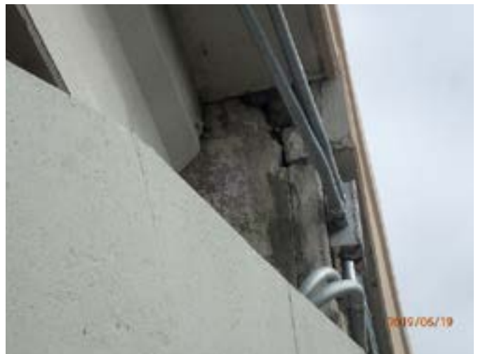
Figure 11: DNT backwall cracking NB at Alpha Road
