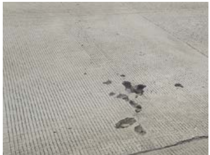
Figure 18: PGBT pavement spalling
