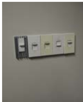
Figure 52: Gleneagles 5900 cover plate missing from light switch
