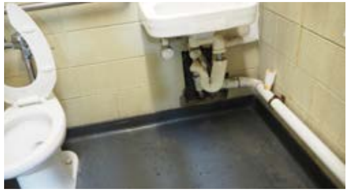
Figure 49: OHIO hole in wall at sink plumbing
