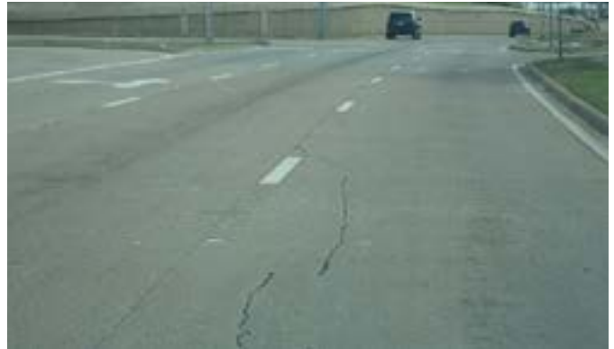
Figure 32: SRT pavement cracking NBFR at MacArthur Boulevard
