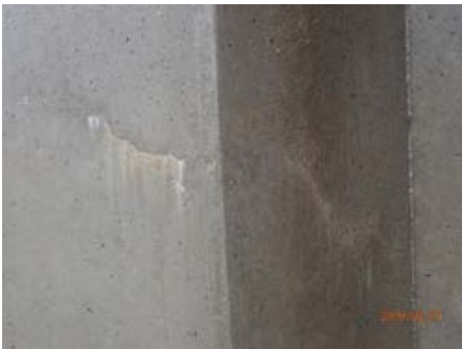
Figure 43: CTP backwall cracking
