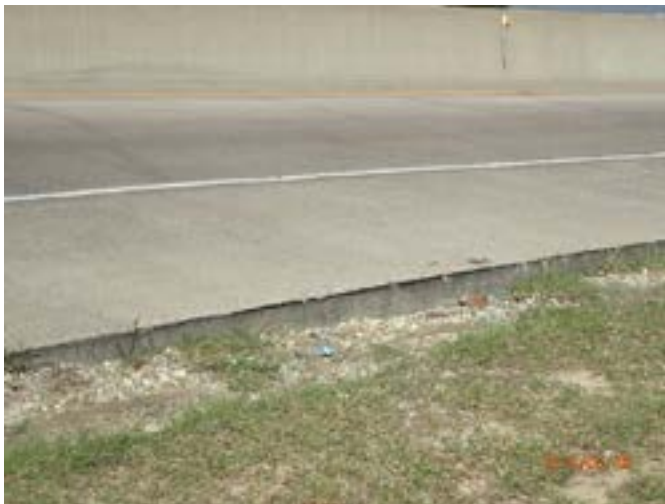
Figure 4: DNT pavement edge drop off
