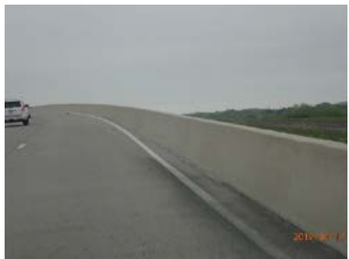
Figure 14: PGBT missing delineation
