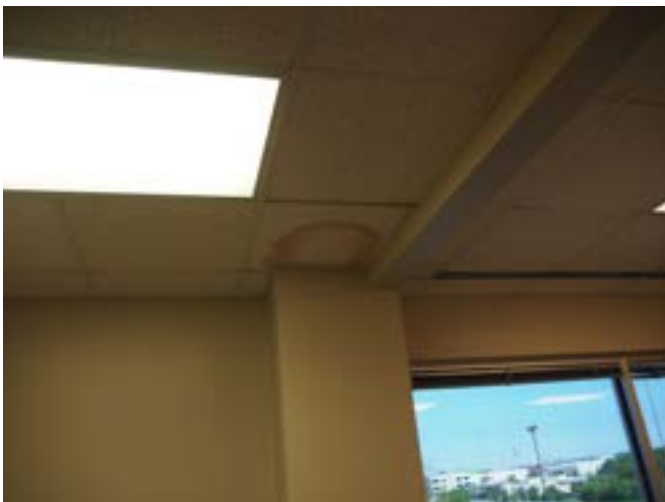
Figure 25: PGBT MLP07 stain on ceiling indicating leak
