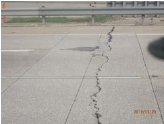
Figure 17: PGBT pavement cracking
