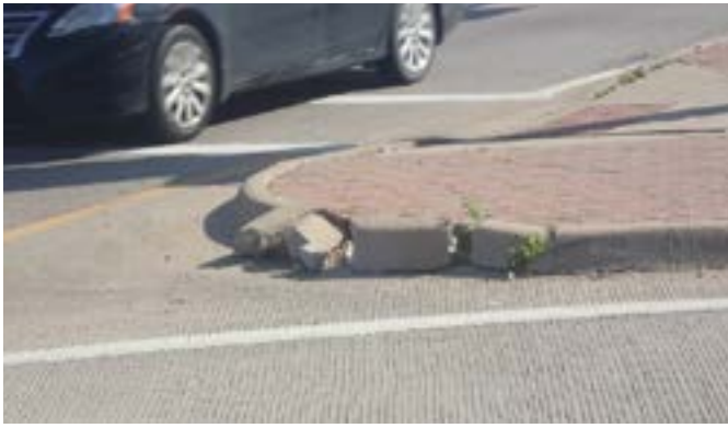
Figure 29: SRT curb damage
