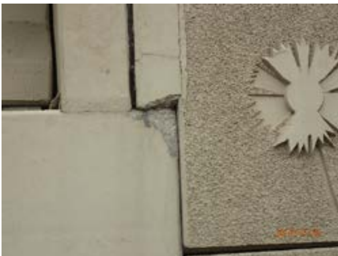
Figure 19: PGBT wall spall with exposed steel
