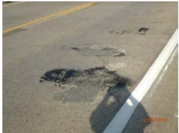
Figure 45: MCLB pavement failure in deck surface treatment
