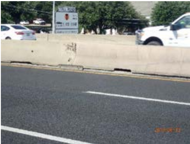
Figure 2: DNT barrier wall spall NB south of Trinity Mills Road
