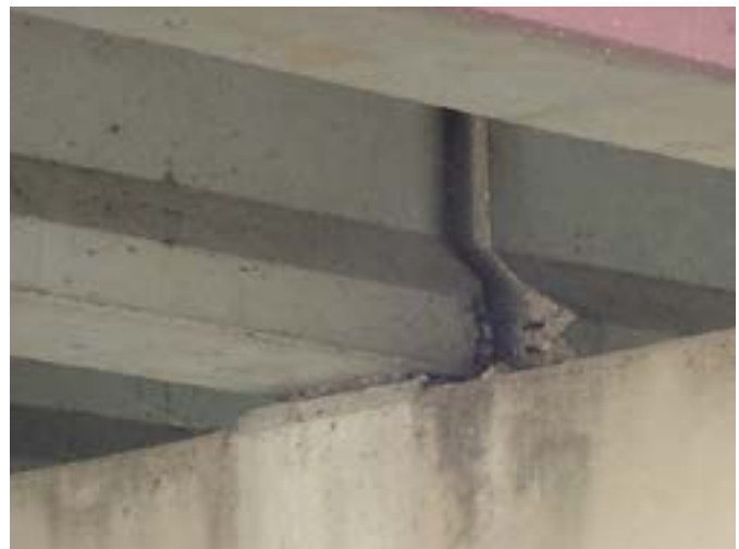
Figure 46: MCLB beam spalling with exposed steel at bent 12
