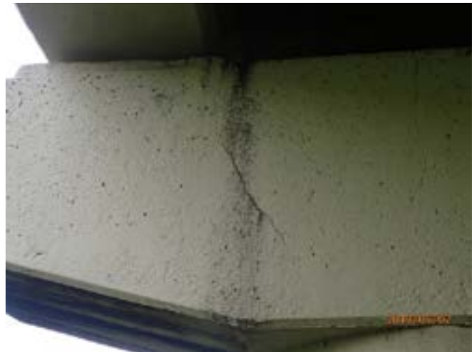
Figure 24: PGBT minor bent cap cracking at Brand Road
