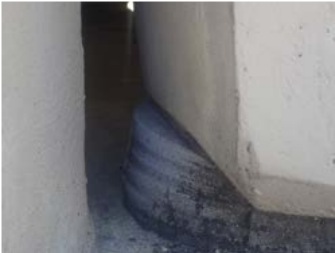
Figure 21: PGBT bearing pad movement
