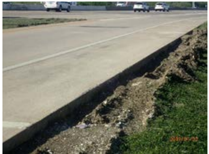
Figure 28: SRT pavement edge drop off
