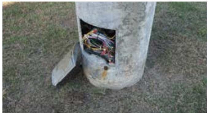
Figure 50: FRISCO cover plate missing from pull box
