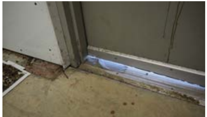
Figure 36: SRT MLG2 gap at door threshold
