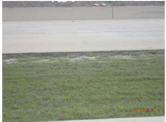
Figure 16: PGBT pavement edge drop off
