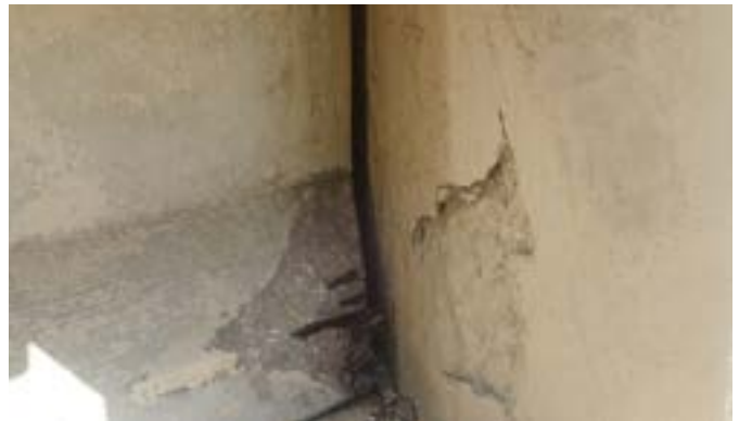
Figure 34: SRT beam and backwall spalling NBFR relief bridge
