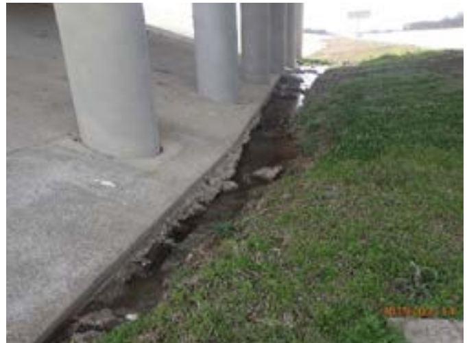
Figure 38: CTP erosion at riprap toe
