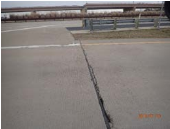
Figure 41: CTP pavement joint damage
