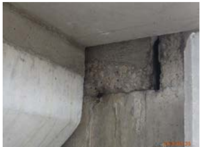
Figure 20: PGBT abutment backwall spall NB at Rowlett Creek
