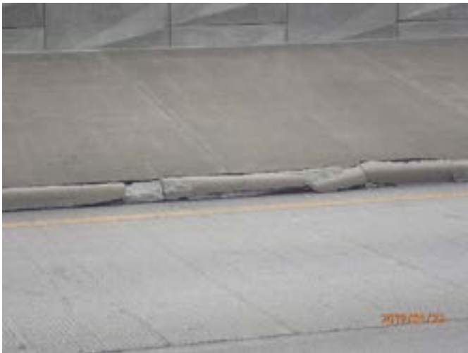
Figure 15: PGBT damaged curb
