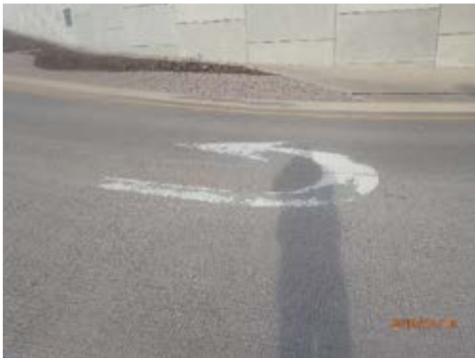
Figure 27: SRT faded pavement markings
