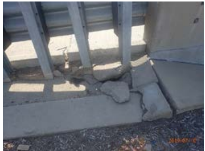
Figure 5: DNT MBGF foundation cracking SB north abutment at Main Street
