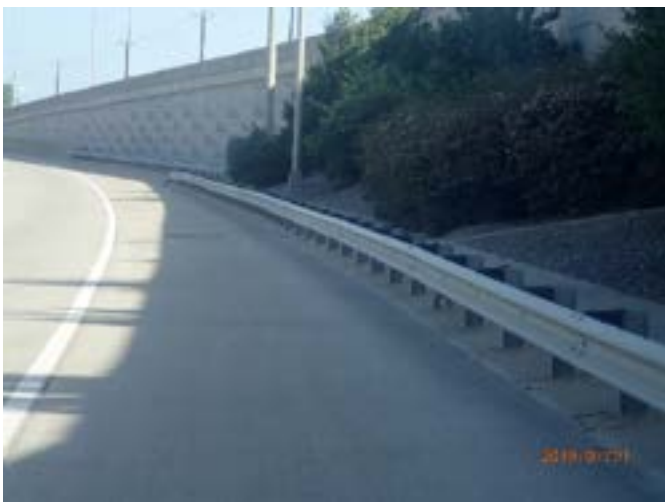
Figure 6: DNT delineation missing on MBGF NB north of Stonebrook Parkway
