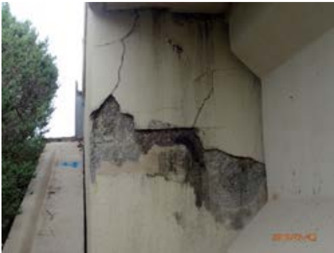
Figure 23: PGBT back wall cracking and spalling at Brand Road
