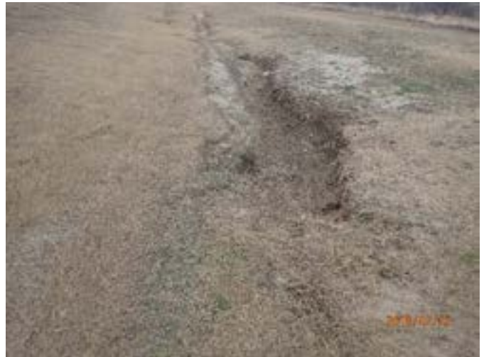
Figure 40: CTP erosion in ditchline
