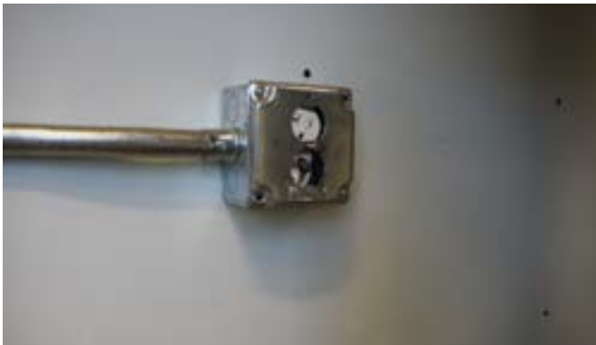
Figure 35: SRT MLG1 electrical outlet damage
