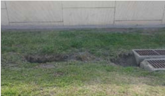
Figure 31: SRT erosion at drop inlet NBML at Old Denton Road
