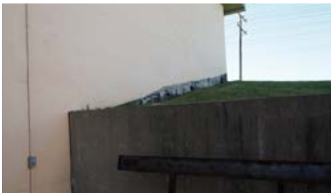
Figure 48: OHIO soil settlement along wall
