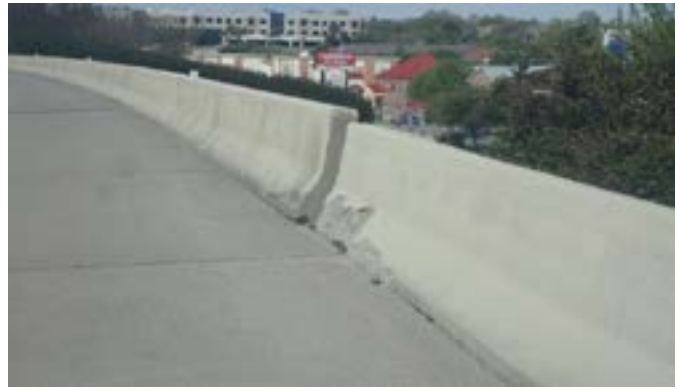
Figure 30: SRT Barrier spall SB South of MacArthur Boulevard
