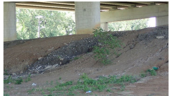
Figure 22: PGBT erosion around columns at Lower Tarrant Road
