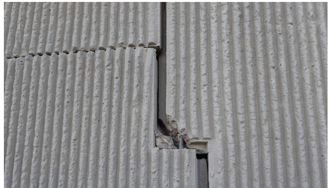
Figure 8: DNT retaining wall panel spall SB at Alpha Rd.
