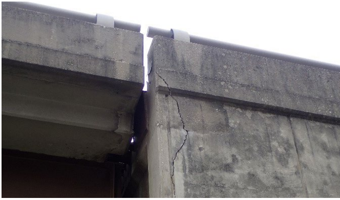
Figure 11: DNT bridge abutment cracking at Harry Hines
