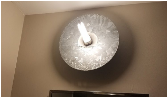
Figure 23: PGBT MLP06 lens missing from light fixture
