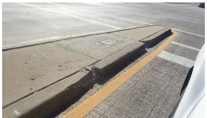
Figure 45: MCLB curb damage on east end
