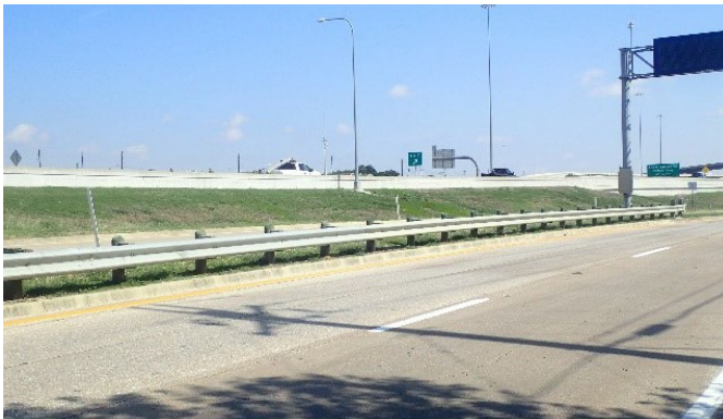
Figure 14: PGBT missing delineation south of Tarrant Rd.
