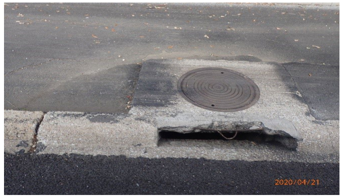
Figure 7: DNT curb inlet damage with steel exposed SB north of Bordeaux
