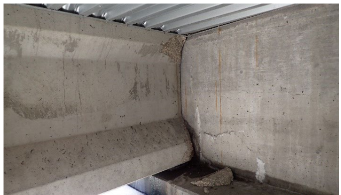
Figure 10: DNT beam spall and touching backwall NB at Main St.
