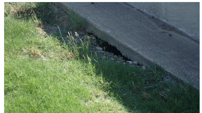
Figure 15: PGBT erosion under mow strip at Oakdale Rd.
