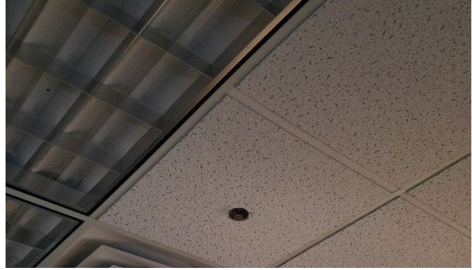
Figure 52: Gleneagles 5900 sprinkler head missing
