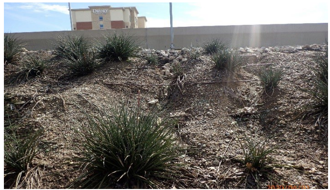
Figure 3: DNT planting bed erosion at Gaylord Parkway
