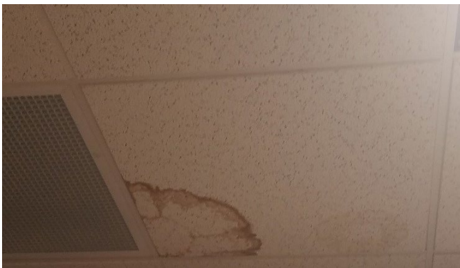
Figure 49: Ohio stain on ceiling indicating leak
