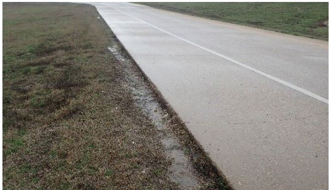
Figure 39: CTP pavement edge drop off SB ramp to FM 1902
