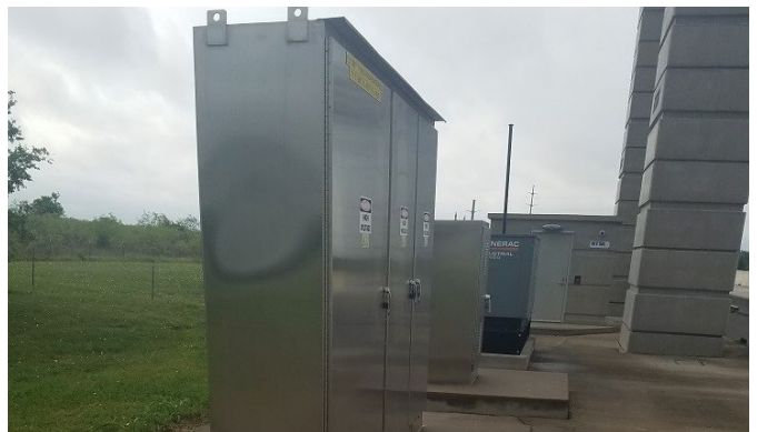
Figure 44: CTP MLP3 cabinet leaning and sealant failing due to settlement
