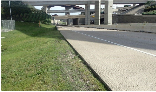
Figure 16: PGBT pavement edge dropoff west of Tarrant Rd.
