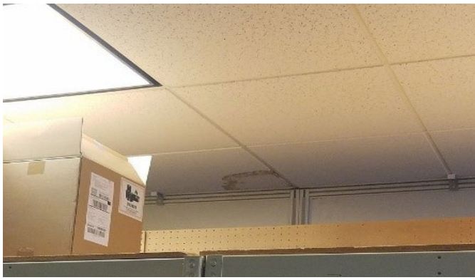
Figure 53: Gleneagles 5910 water-stained ceiling tiles
