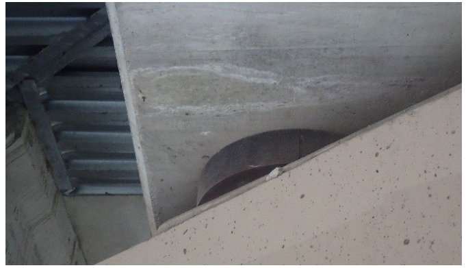
Figure 42: CTP bearing pad movement at relief bridge north of Hulén St.
