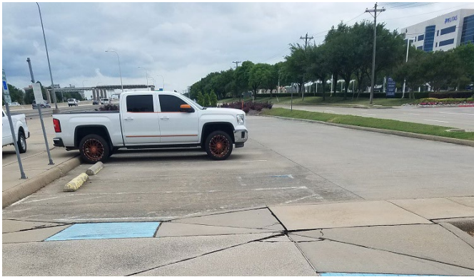
Figure 12: DNT MLP3 – pavement paint faded
