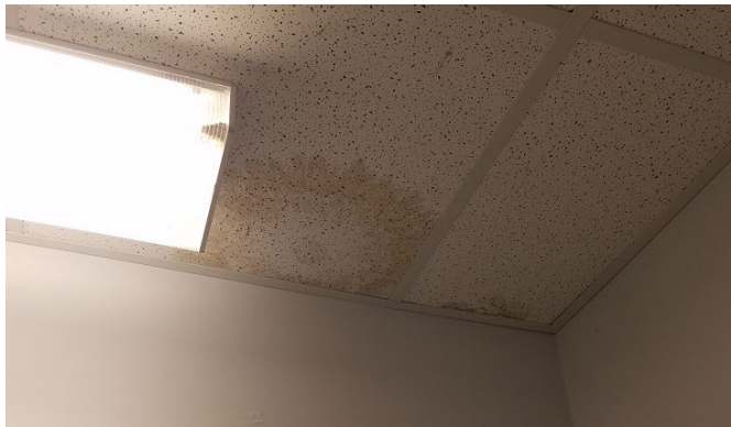
Figure 13: DNT MLP4 – stains on ceiling tile
