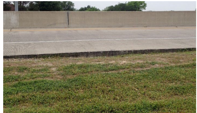
Figure 4: DNT pavement edge dropoff SB to WB IH-635
