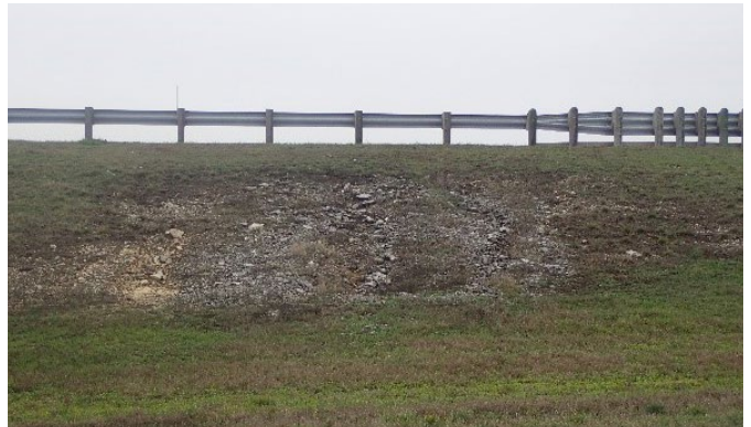
Figure 38: CTP embankment erosion at NB ramp from FM 1187
