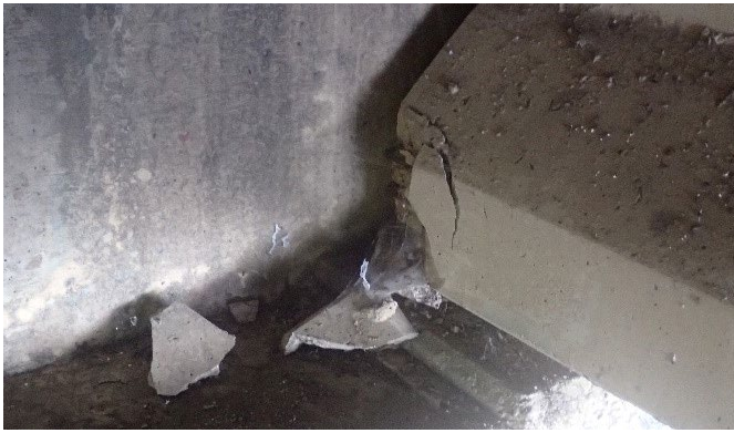
Figure 46: MCLB beam end spalling at west abutment
