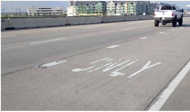
Figure 27: SRT faded striping SB ramp to Standridge Dr.
