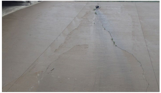
Figure 37: CTP riprap cracking at FM 917
