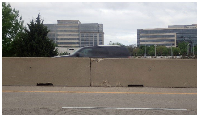
Figure 2: DNT barrier wall spall NB north of Gaylord Pkwy
