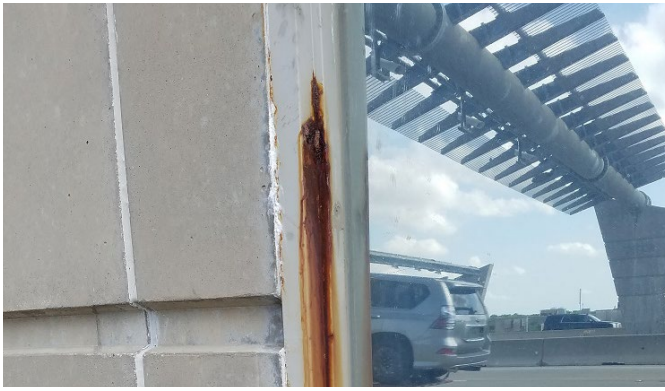
Figure 35: SRT MLG02 rust development at window frame
