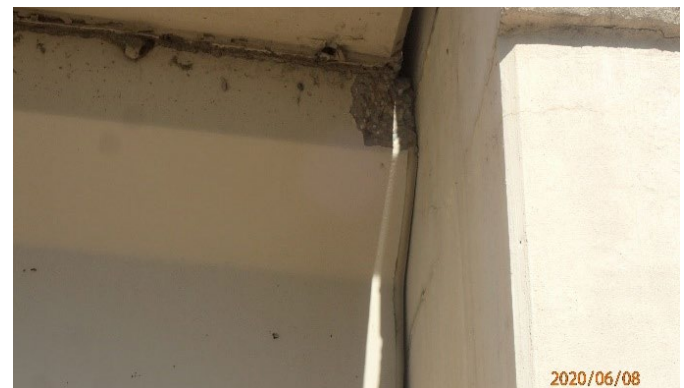
Figure 21: PGBT beam end spall at IH-30
