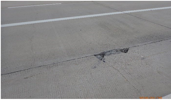
Figure 41: CTP pavement spall NB north of FM 1187
