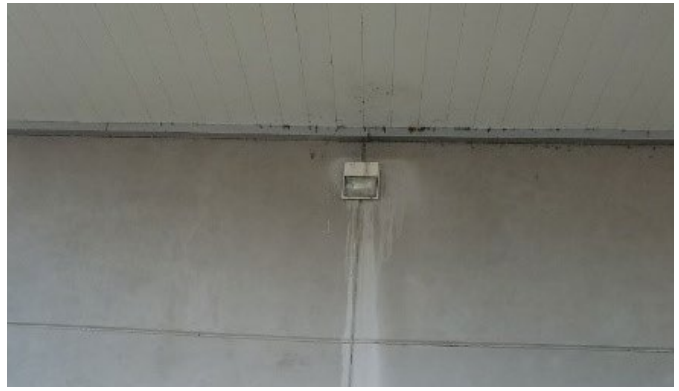
Figure 50: Frisco water intrusion into light fixture
