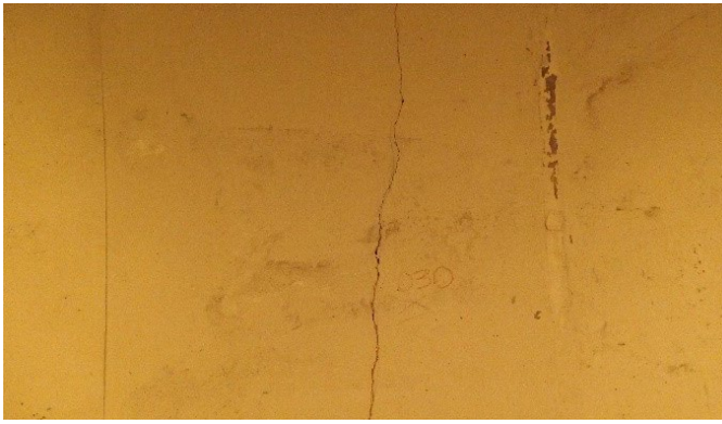
Figure 47: AATT wall cracking at multiple locations
