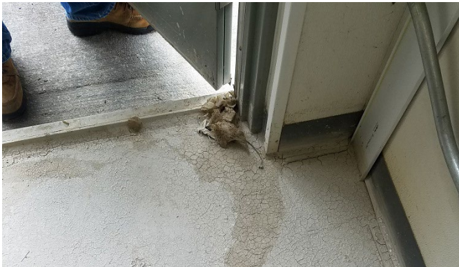
Figure 36: SRT MLG03 water intrusion into building
