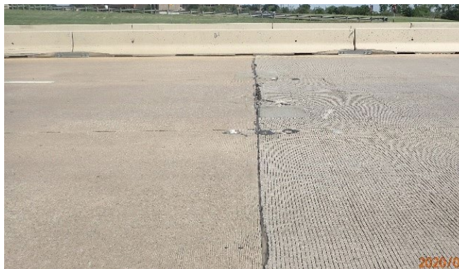
Figure 18: PGBT pavement spall north of Las Colinas
