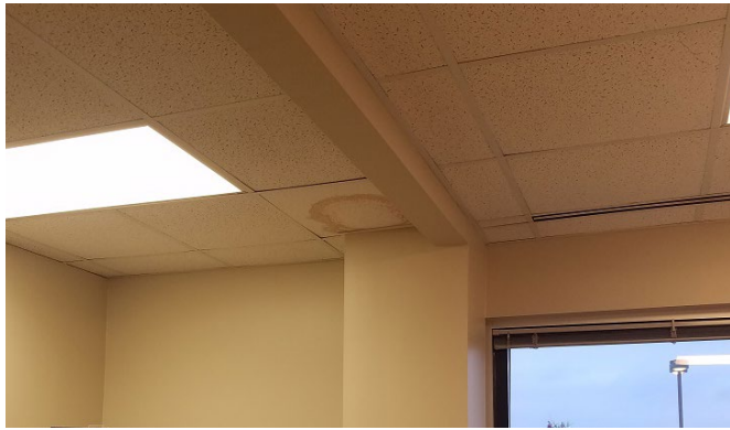
Figure 24: PGBT MLP07 stains on ceiling tile
