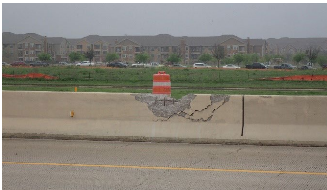
Figure 30: SRT barrier wall damage NB at Carrollton Pkwy.
