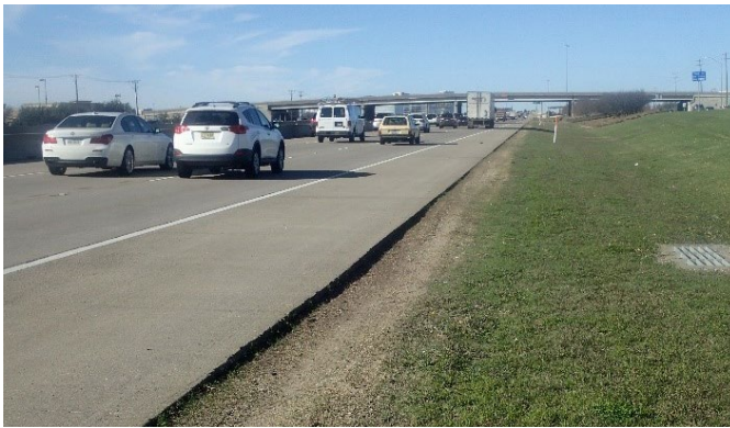
Figure 28: SRT pavement edge dropoff SB ramp to Stacy Rd.
