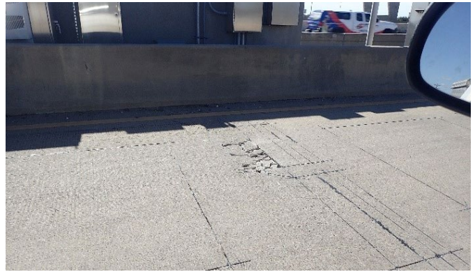
Figure 32: SRT pavement spall SB from Ohio Dr.
