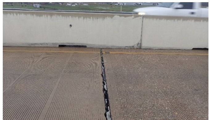
Figure 40: CTP pavement joint seal deterioration SB south of CR 1016
