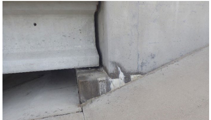
Figure 43: CTP backwall cracking SB south of CR 913
