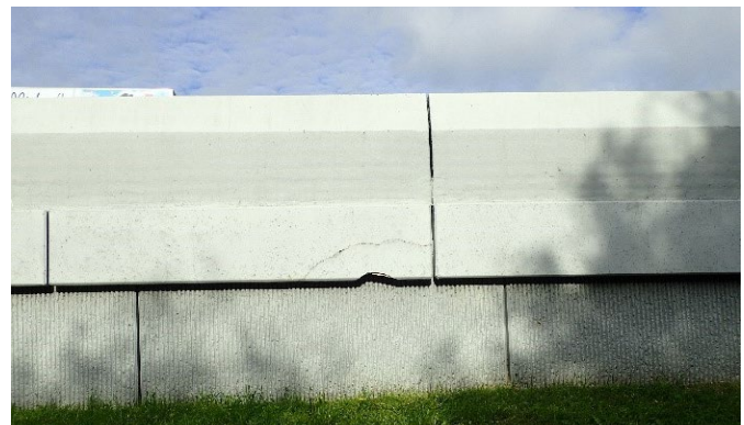
Figure 9: DNT wall coping cracking and spalling SB SRT to NB DNT
