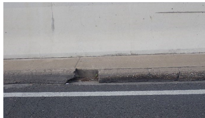
Figure 5: DNT curb spall NB south of University Blvd.
