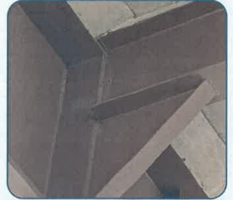
Figure 122: DNT SB to IH-35E – Fracture Critical Weld Repairs.
