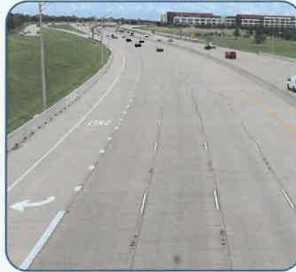
Figure 129: SRT near FM 544 – Mainlane and Frontage Road Restriping.
