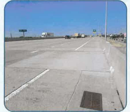
Figure 130: SRT at Plano Pkwy. – Concrete Pavement Repairs.
