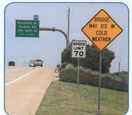
Figure 127: PGBT near Arkansas Ln. – Large and Small Sign Replacement.
