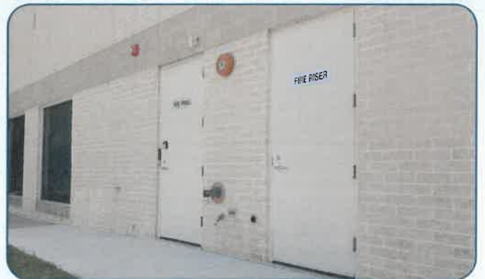
Figure 134: Gleneagles 5900 – Exterior Building Refurbishment.
