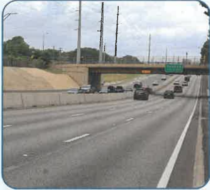
Figure 120: DNT NB near Northaven Rd. – Mill and Overlay.
