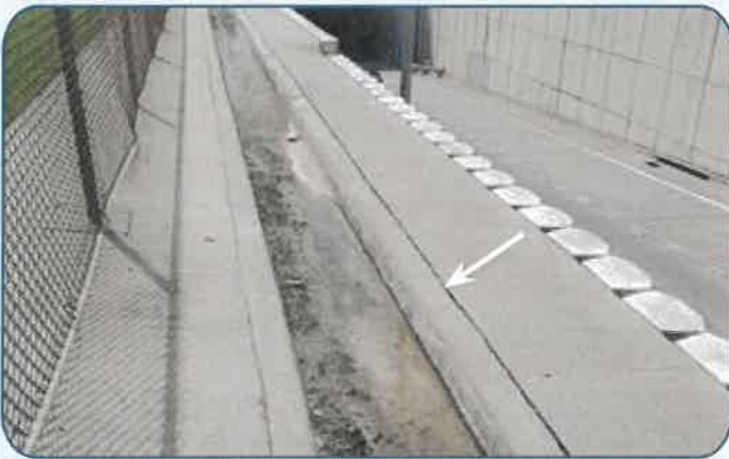
Figure 85: AATT Unsealed Concrete Flume at East End.
