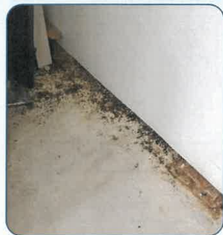
Figure 84: LLTB Fiber Hut Insect Infestation.
