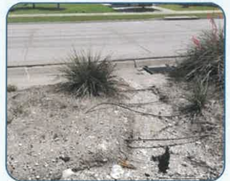
Figure 5: DNT NB Landscape Bed Erosion North of Cotton Gin Rd.
