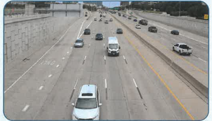
Figure 124: DNT near Tennyson Pkwy. – Restriping.
