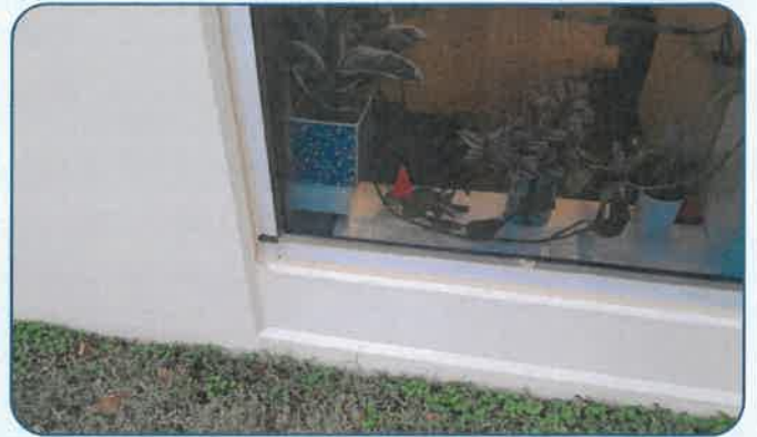
Figure 136: Gleneagles Window Seal Replacement.
