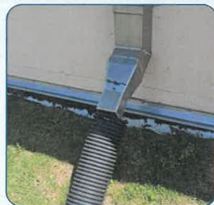
Figure 110: POC Storage Building Separated Roof Drain.
