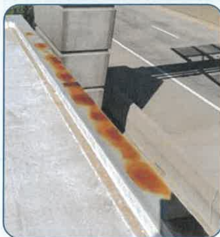
Figure 83: LLTB Fiber Hut Degraded Roof.
