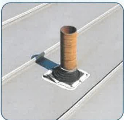
Figure 111: POC Roof Damaged Pipe Penetration.
