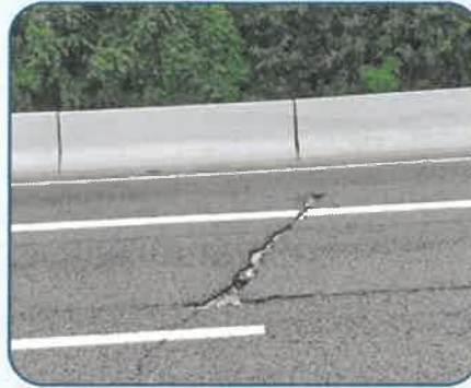
Figure 2: DNT SB Reflective Pavement Cracking South of Galleria Dr.
