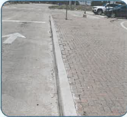
Figure 128: SRT near Legacy Dr. – SRT Curb Repairs.
