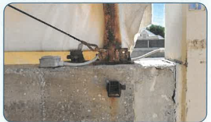
Figure 19: DNT Meaders Lane Winter Weather Operations Facility Corroded Member.
