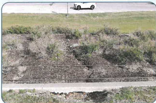
Figure 39: SRT WB Landscape Bed Erosion East of Legacy Dr.
