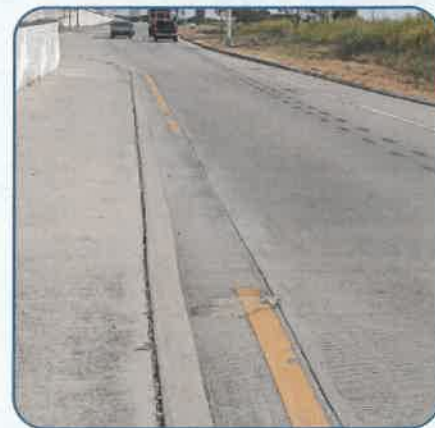
Figure 22: PGBT SB Damaged or Faded Pavement Markings North of Merritt Rd.
