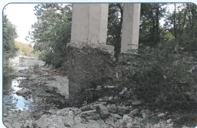
Figure 29: PGBT Exposed Column Footings at US 75.
