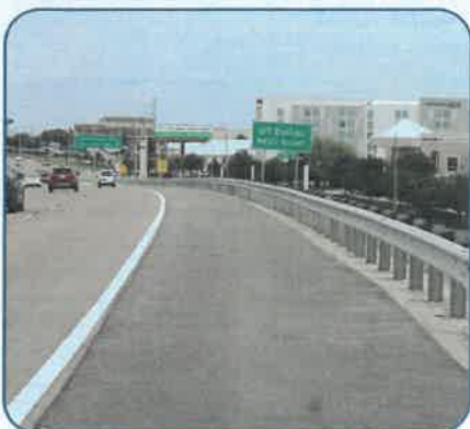
Figure 125: PGBT near Coit Rd. – Mill and Overlay Outside Shoulder.
