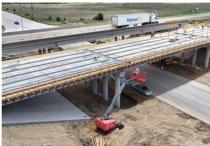
Prepping for concrete placement at CR 920
