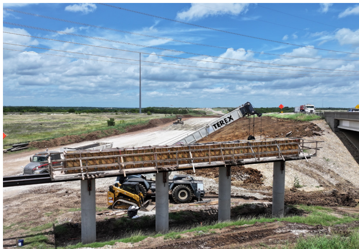
Concrete placement for cap at CR 1016
