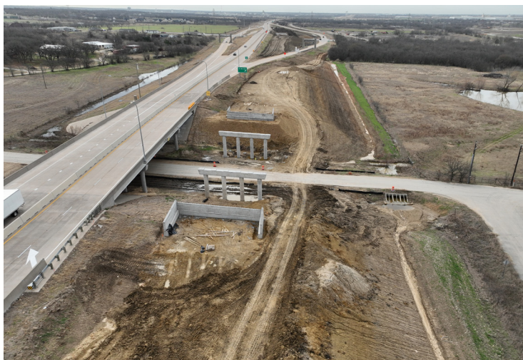
Column and cap construction at Don Lee Rd.
