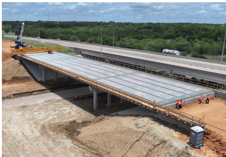
Deck work at Don Lee Rd.
