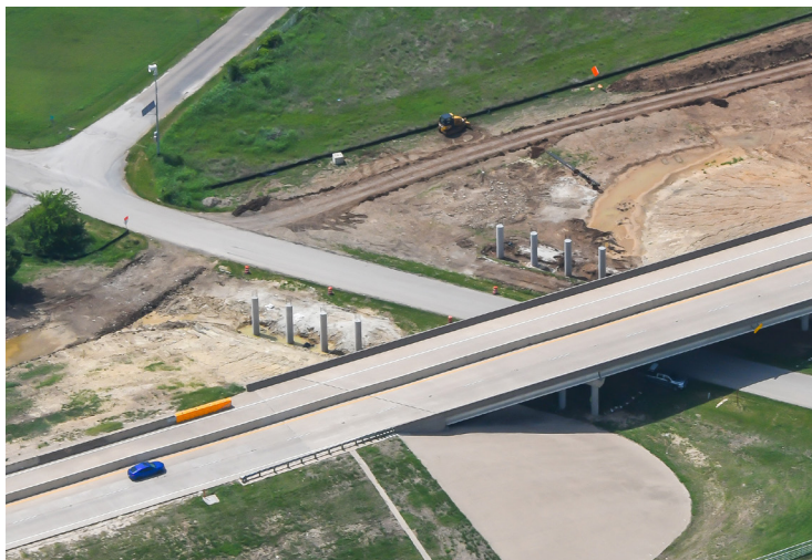
Column construction at CR 1016
