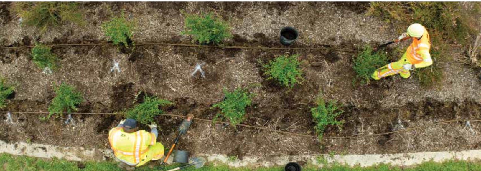
Landscape crew placing new shrubs along SRT
