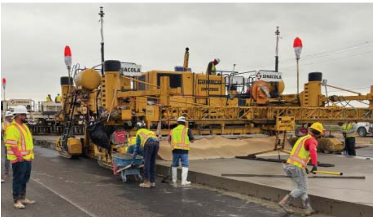
Placing concrete for southbound mainlanes
