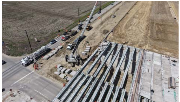
Placing deck panels at Punk Carter Pkwy.
