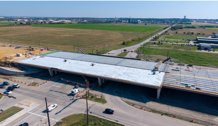
Deck work at First St.
