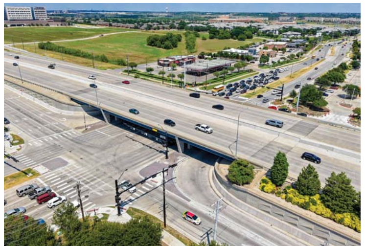
Additional lanes open over Eldorado Pkwy. intersection
