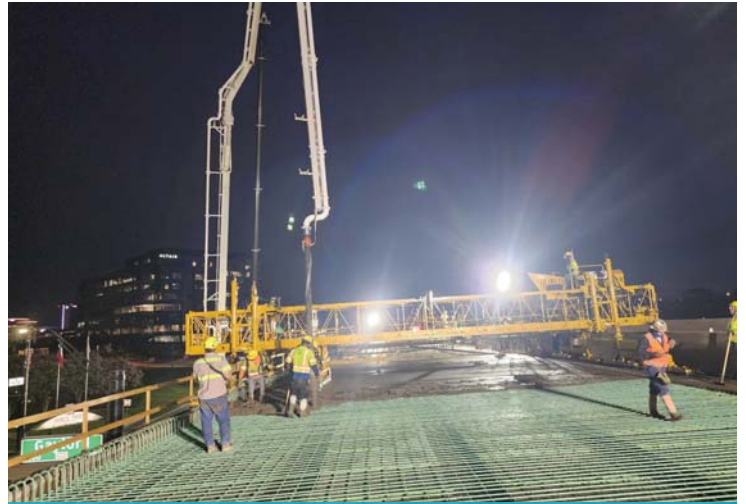
Concrete placement for bridge widening over Gaylord Pkwy.
