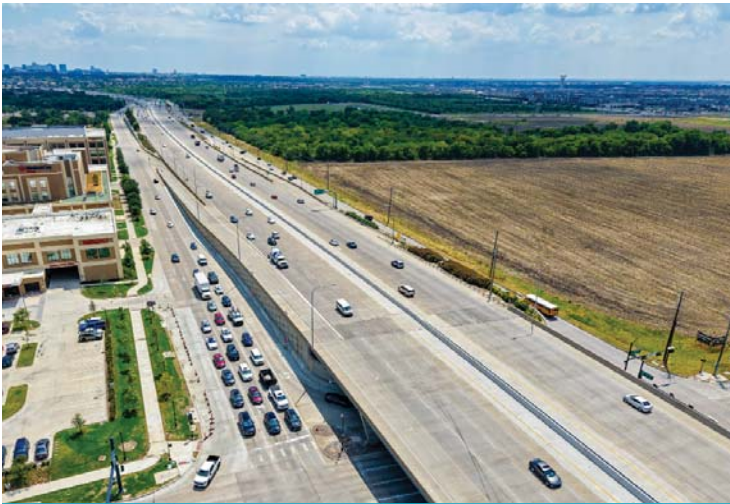
Additional lanes opened to traffic
