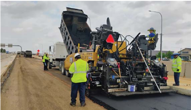
Subgrade placement for shoulder
