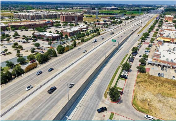
New ramps at Main St. and Eldorado Pkwy. opened to traffic in late July
