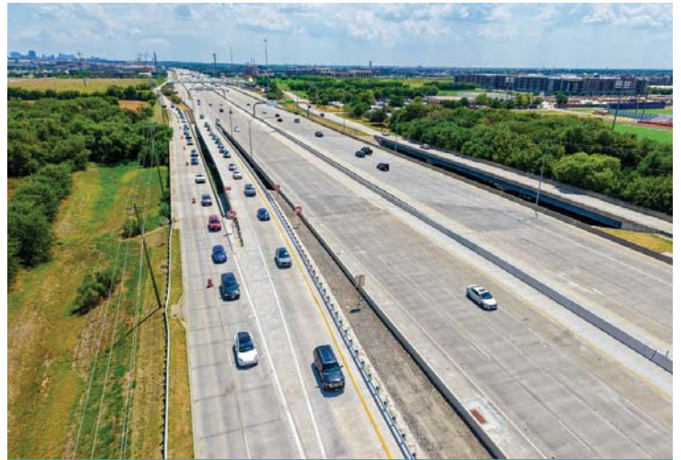
The new northbound Eldorado Pkwy. exit ramp opened to traffic in late July
