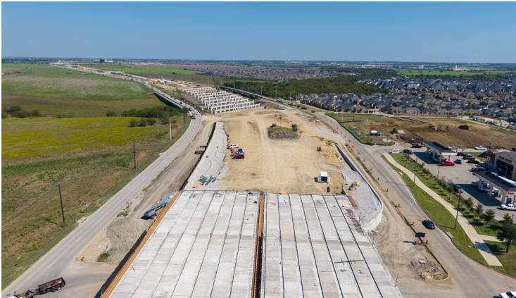
Deck and column work at Light Farms Way and Doe Branch Creek
