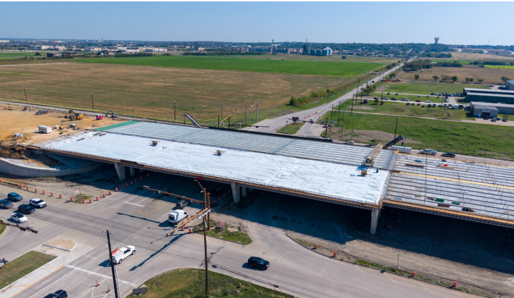
Deck work at First St.
