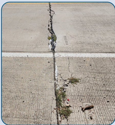
Figure 54: CTP SB Pavement Joint Deterioration North of Arborlawn Dr.
