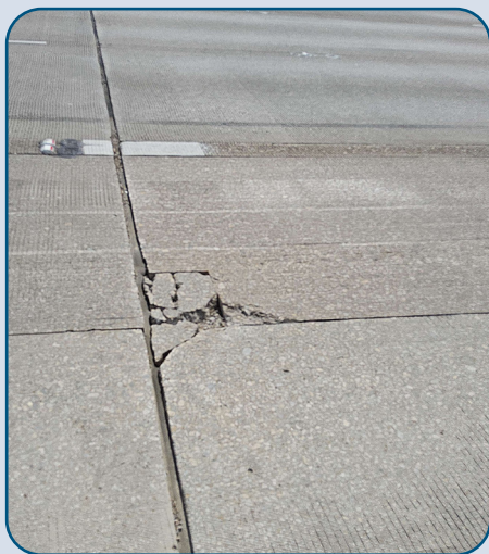
Figure 39: SRT WBML Pavement Spalling West of Hillcrest Rd.
