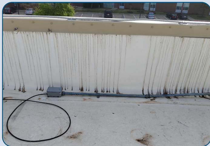
Figure 34: MLP6 Roof Coping Degradation.
