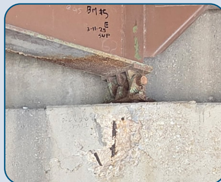
Figure 13: DNT Abutment Spalling at Lomo Alto Dr.
