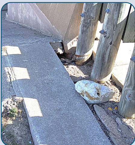
Figure 62: CTP SB Erosion and Undermining of MBGF Mow Strip and Adjacent Concrete Riprap South of McPherson Blvd.
