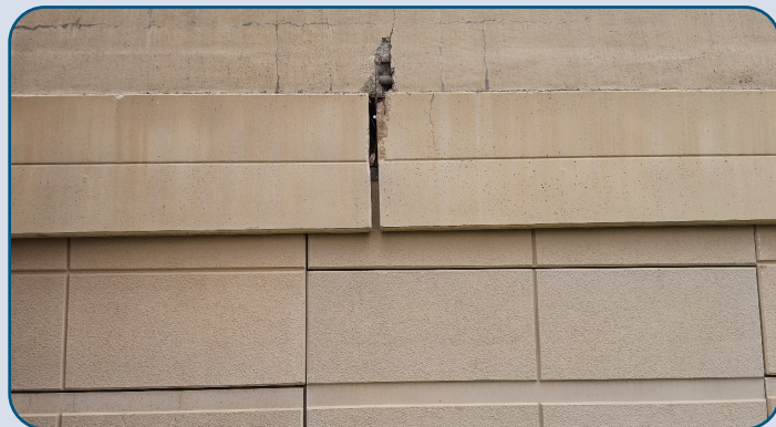
Figure 61: CTP MSE Wall Coping and Concrete Rail Spalling South of Overton Ridge Blvd.
