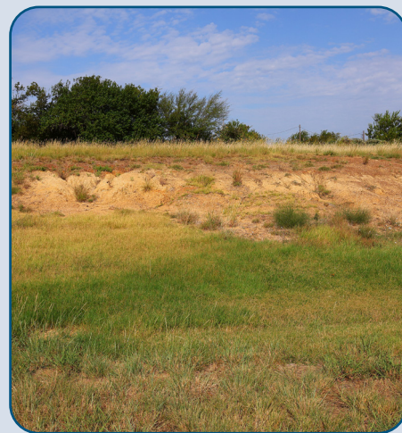
Figure 59: CTP SB Turf Erosion South of CR 913.
