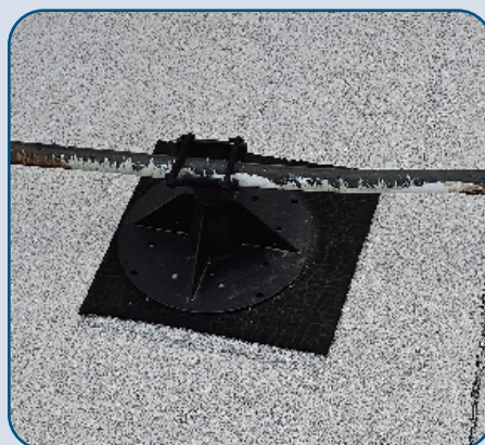
Figure 117: Gleneagles 5900 Bent HVAC Drain Pipe.
