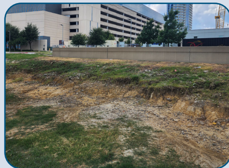
Figure 4: DNT NB Turf Erosion South of SRT.
