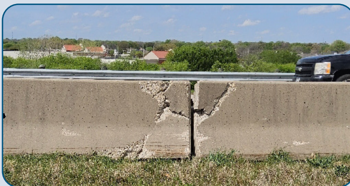
Figure 99: 360T SB Concrete Rail Cracking and Spalling South of SE Green Oaks Blvd.
