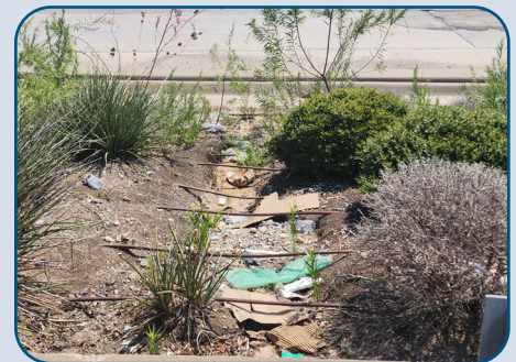
Figure 5: DNT NB Landscape Bed Erosion North of Main St.
