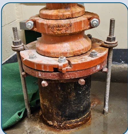
Figure 110: POC Fire Riser Corrosion.
