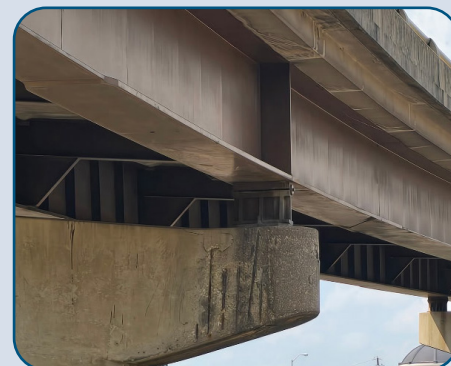
Figure 14: DNT Bent Cap Spalling North of IH 35E.
