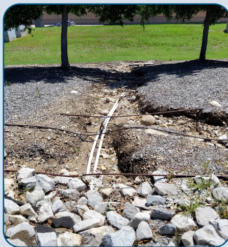
Figure 58: CTP NB Landscape Bed Erosion with Exposed Irrigation South of IH 20.
