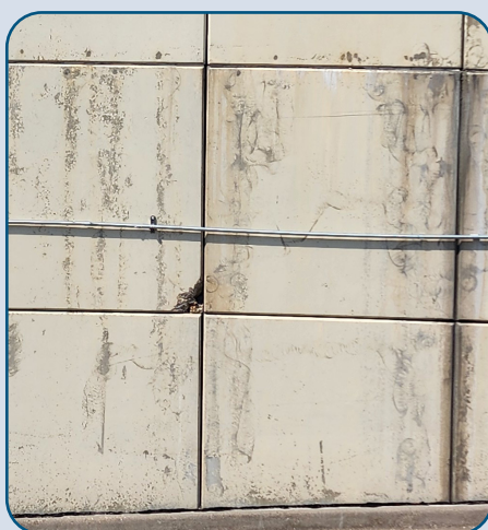
Figure 89: AATT Panel Wall Spalling.
