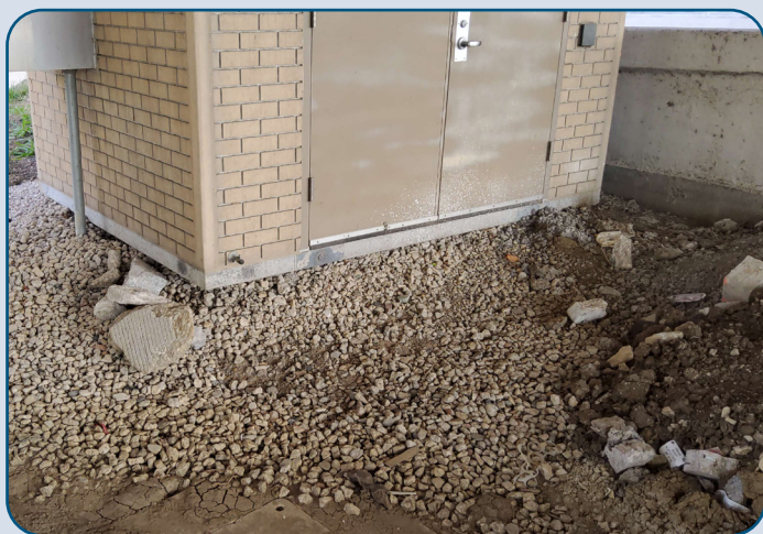
Figure 35: PGBT Fiber Hut 5 Erosion.
