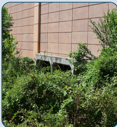
Figure 63: CTP NB Obstructions at Bridge Class Culvert Headwall North of Dutch Branch Rd.
