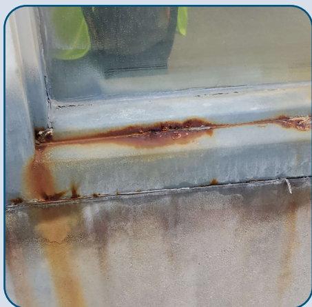
Figure 15: DNT MLG1 Window Frame Corrosion.
