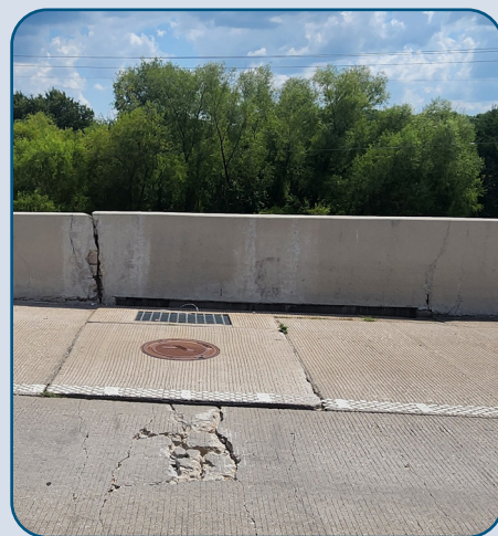
Figure 23: PGBT NB Concrete Rail Cracking and Spalling North of Miller Rd.
