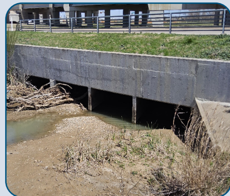
Figure 103: 360T SB Bridge Class Culvert with Sediment Buildup and Obstructions South of Lone Star Rd.
