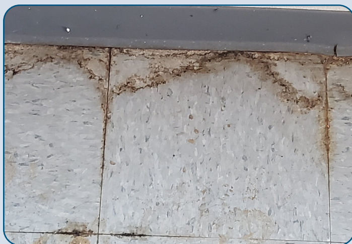
Figure 66: CTP MLG2 Water Infiltration.
