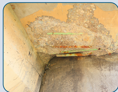
Figure 48: SRT NB Under Deck Spalling West of Spring Creek Pkwy.
