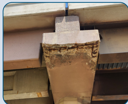
Figure 12: DNT Bent Cap Spalling at IH 635.
