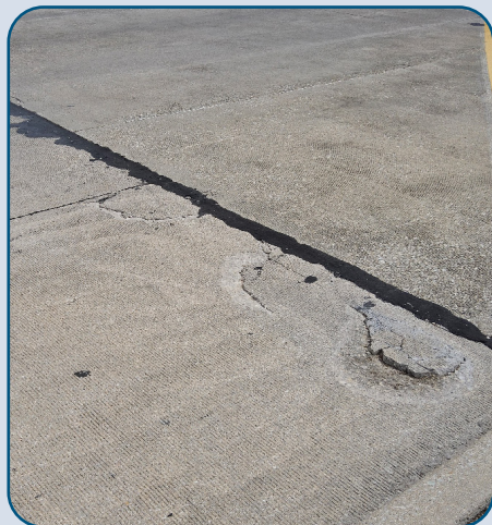
Figure 86: AATT Pavement Spalling.
