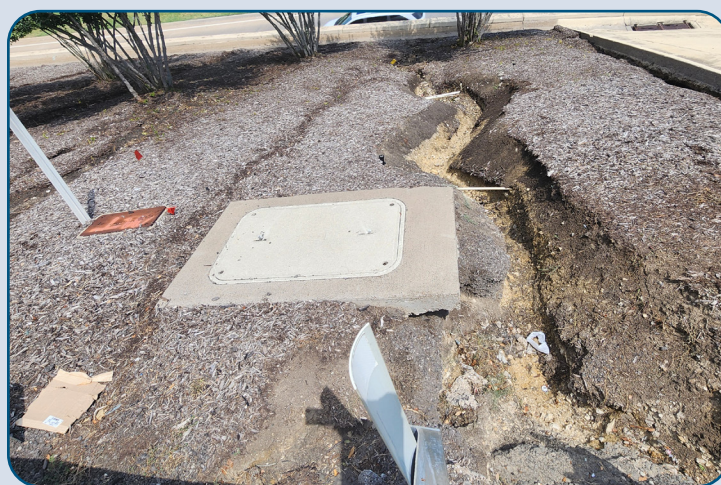
Figure 25: PGBT WB Landscape Bed Erosion at Coit Rd.
