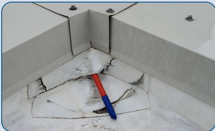
Figure 51: SRT MLG1 Damaged Roof.
