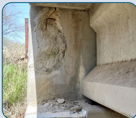
Figure 104: 360T SB Backwall Cracking and Spalling North of N. Holland Rd.
