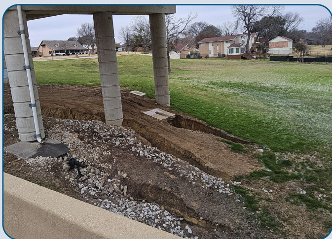
Figure 24: PGBT SB Slope Erosion North of IH 30 in Garland.
