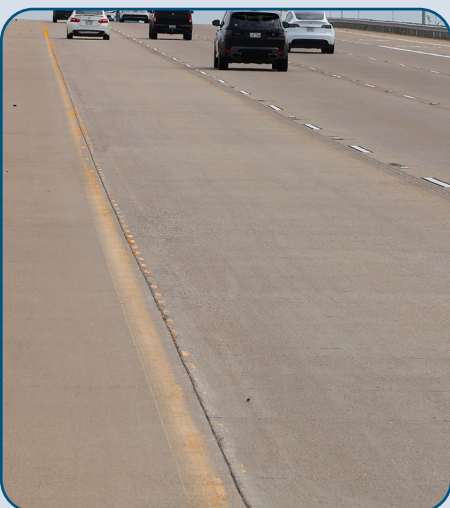
Figure 42: SRT EBML Faded Pavement Markings West of Stacy Rd.
