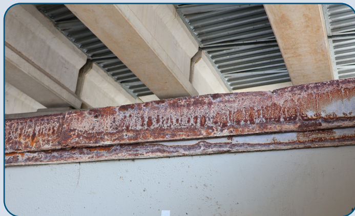
Figure 52: SRT Restroom Corroded Roof.
