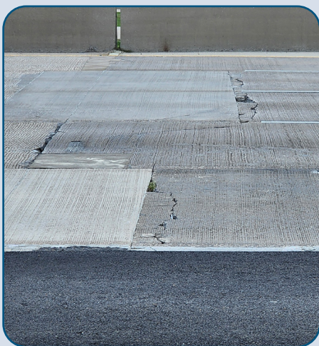
Figure 21: PGBT WB Pavement Cracking and Spalling West of Alma Rd.
