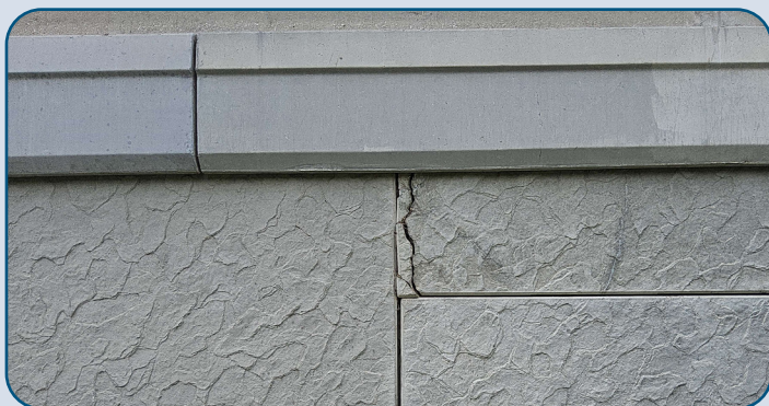
Figure 100: 360T NB MSE Wall Panel Cracking North of N. Holland Rd.
