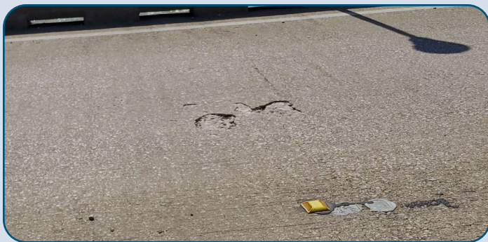
Figure 71: MCLB Deck Spalling.
