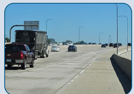
Figure 7: DNT NB Faded Pavement Markings North of PGBT.
