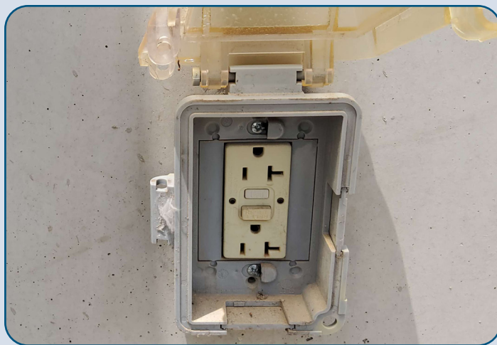
Figure 107: 360T MLG15 Electrical Receptacle Failure.
