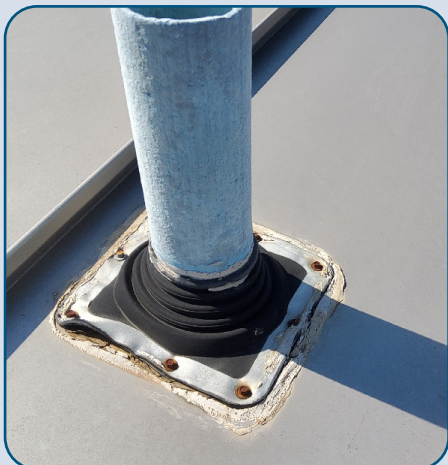
Figure 113: POC Damaged Roof Penetration.
