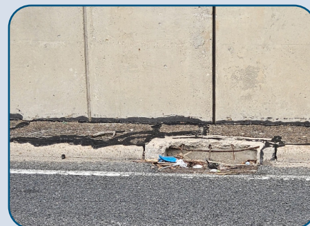
Figure 6: DNT NB Inlet Damage Near Oak Lawn Ave.
