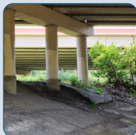
Figure 30: PGBT Channel Erosion at White Rock Creek.
