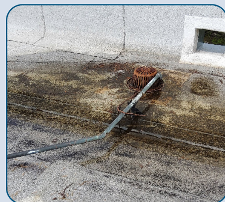
Figure 118: Gleneagles 5900 Deteriorated Roof.
