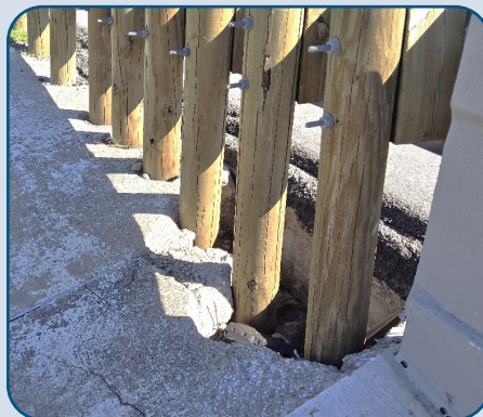
Figure 102: 360T SB MBGF Mow Strip Undermining at SE Green Oaks Blvd.
