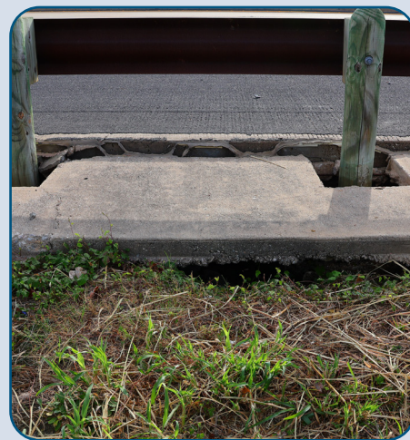
Figure 56: CTP SB Unsealed Joint Undermining Mow Strip South of Dutch Branch Rd.
