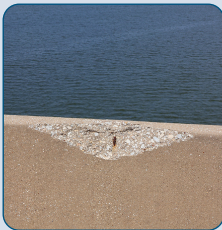
Figure 81: LLTB Concrete Rail Spalling.
