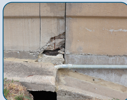
Figure 49: SRT NB Cracked Approach Rail Allowing Water to Erode the Backside at Standridge Dr.
