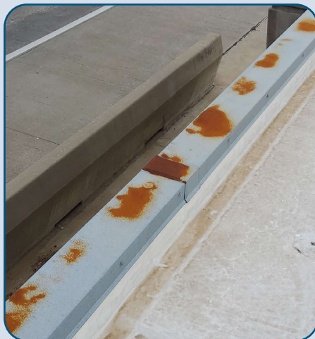
Figure 84: LLTB Fiber Hut Roof Degradation.
