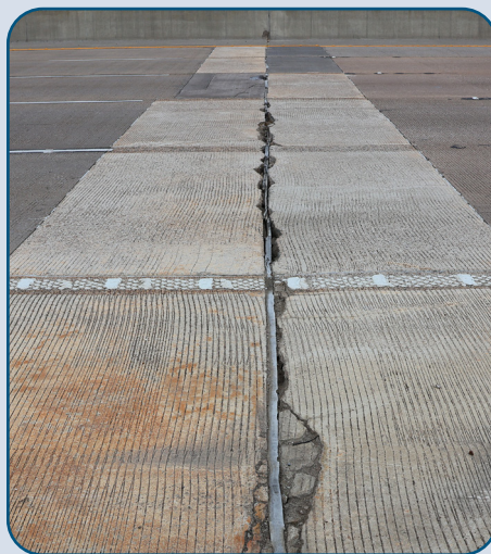
Figure 40: SRT EBML Pavement Joint Deterioration West of Standridge Dr.
