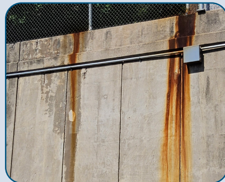
Figure 10: DNT SB Wall Staining at University Blvd.
