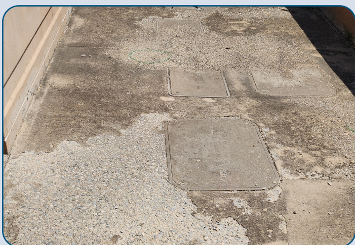
Figure 67: CTP MLG1 Deteriorated Landing.
