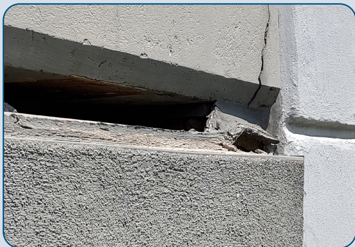
Figure 33: PGBT Midway Road On-Ramp Gantry Panel Separation.
