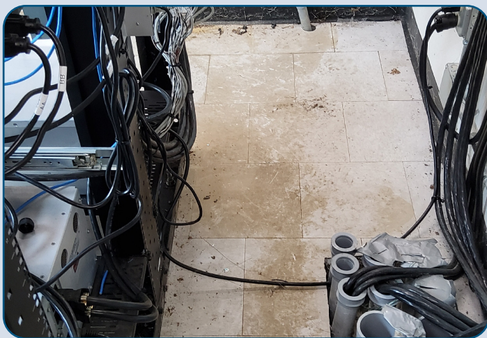
Figure 106: 360T MLG15 Water Infiltration.
