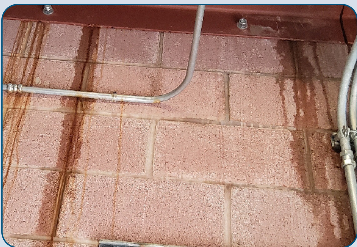
Figure 93: AATT Toll Plaza Electrical Room Water Leak.
