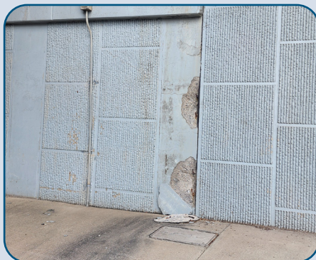
Figure 9: DNT MSE Wall Spalling at Headquarters Dr.
