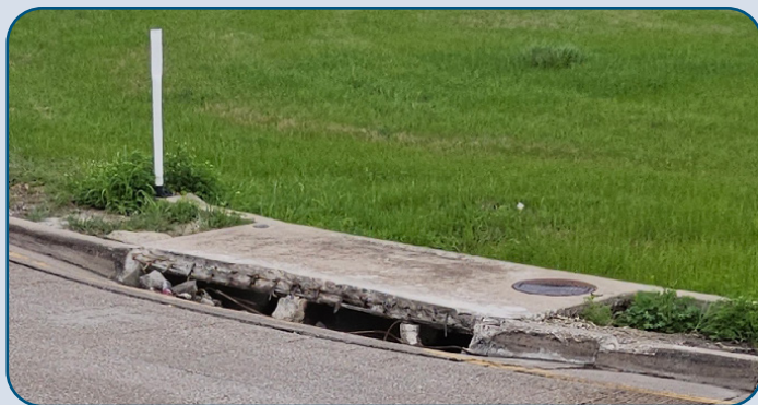
Figure 96: 360T NB Curb Inlet Damage at SE Green Oaks Blvd.
