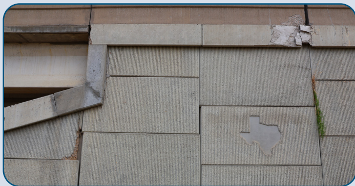
Figure 45: SRT NB MSE Wall Panel and Coping Cracking and Spalling at Spring Creek Pkwy.
