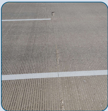
Figure 80: LLTB Deck Spalling.
