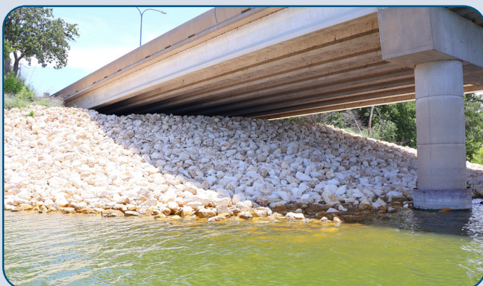
Figure 128: LLTB – Erosion Mitigation East Approach.
