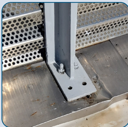
Figure 16: MLP4 Roof Railing Post Partially Reattached.
