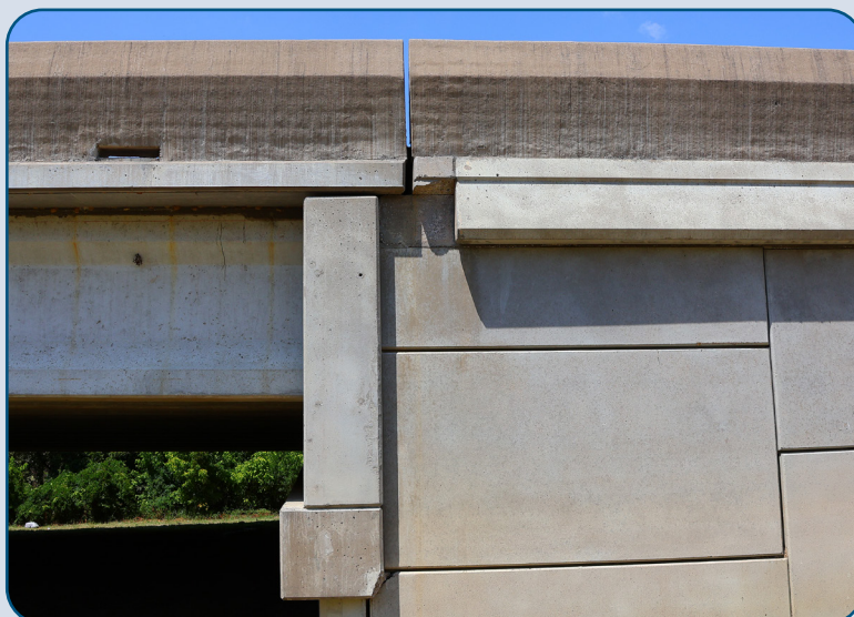
Figure 79: LLTB MSE Wall Coping Damage.
