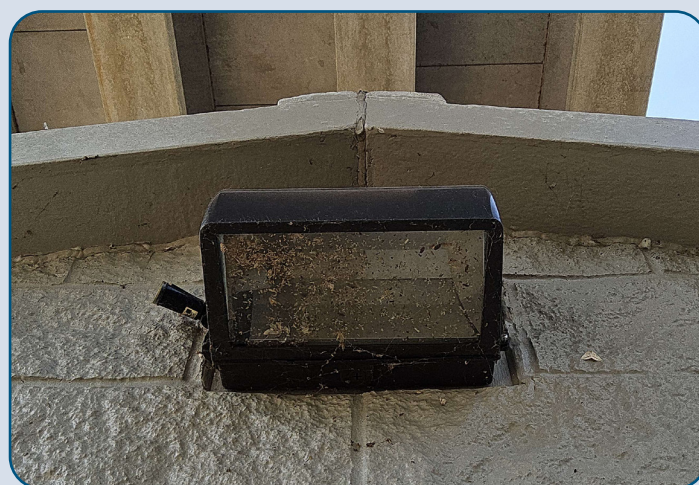
Figure 68: CTP Restroom Light Fixture Insect Infestation.
