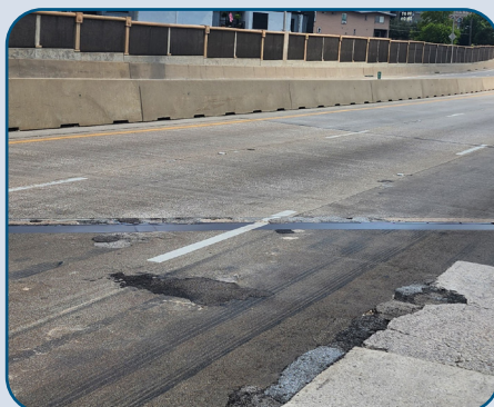
Figure 11: DNT Deck Deterioration at Wycliff Ave.
