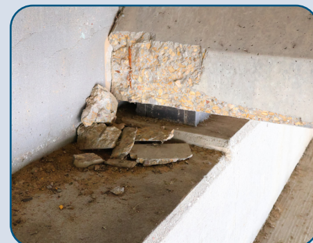
Figure 50: SRT SB Beam Hitting Backwall at West Rowlett Creek.
