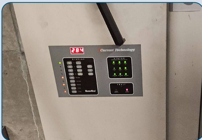
Figure 94: AATT Main Electrical Room Failed Surge Suppressor.
