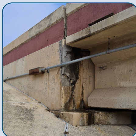
Figure 29: PGBT Backwall Cracking and Spalling West of Hillcrest Rd.
