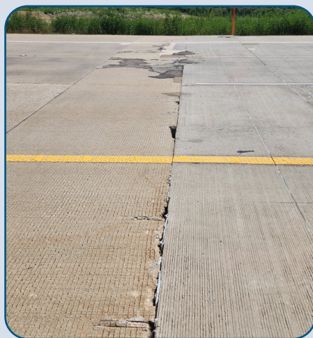
Figure 22: PGBT NB Pavement Joint Deterioration and Spalling North of Merritt Rd.
