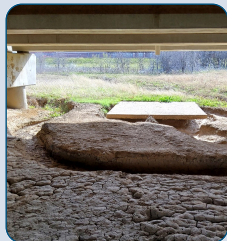
Figure 64: CTP NB Channel Erosion South of CR 913.
