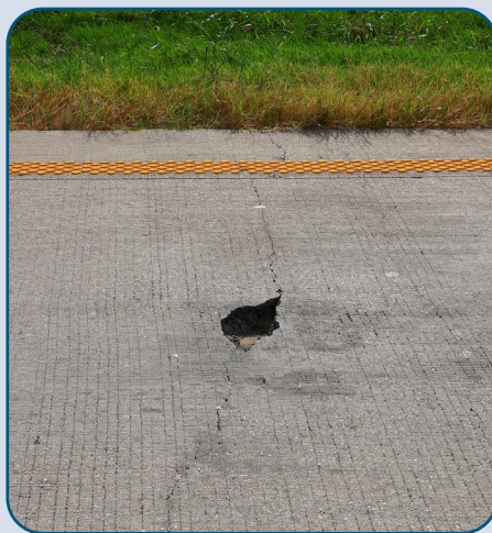
Figure 55: CTP SB Pavement Spalling North of FM 1187.
