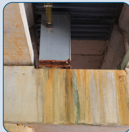
Figure 82: LLTB Corroded Junction Box/Bent Cap Staining.
