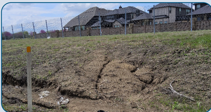
Figure 98: 360T SB Slope Erosion and Sediment Buildup North of Sawmill Way.
