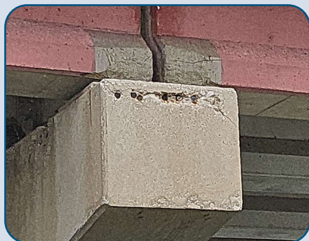
Figure 73: MCLB Bent Cap Spalling with Exposed Reinforcement.
