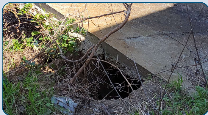
Figure 70: MCLB Storm Sewer Outfall Structure Erosion West End.
