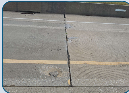
Figure 2: DNT NB Concrete Pavement Spalling North of Eldorado Pkwy.
