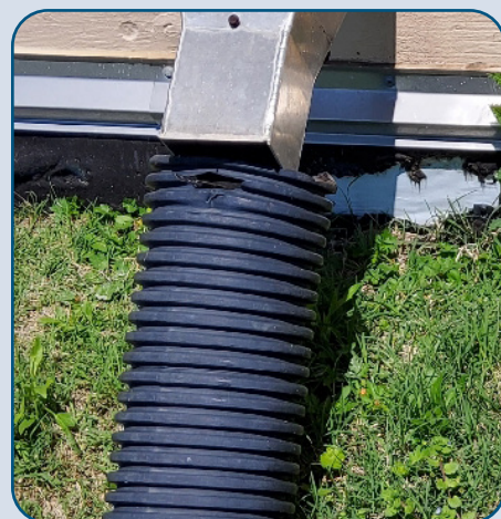
Figure 112: POC Bulk Storage Building Roof Drain Degradation.
