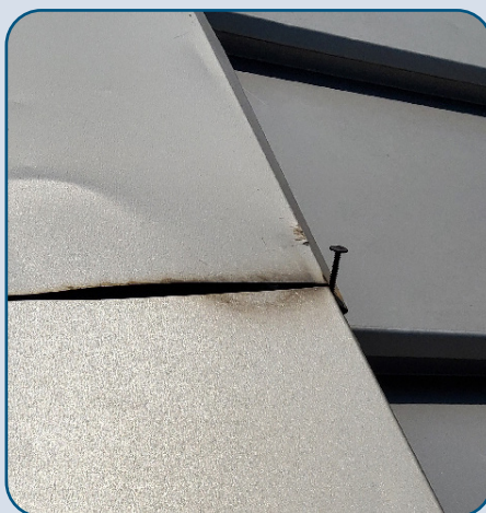
Figure 111: POC Roof Fasteners Loose.
