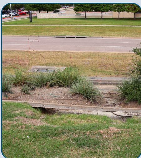
Figure 43: SRT SB Landscape Bed Erosion and Concrete Boarder Undermining West of S. Lake Forest Dr.
