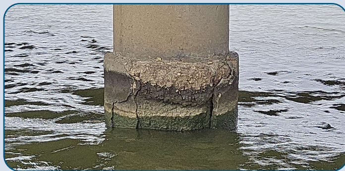
Figure 72: MCLB Column Collars Spalling.
