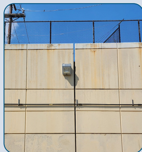
Figure 90: AATT Panel Wall Cracking and Missing Joint Seal.
