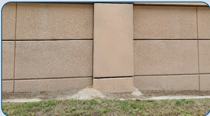
Figure 60: CTP MSE Wall Backfill Migration North of Overton Ridge Blvd.
