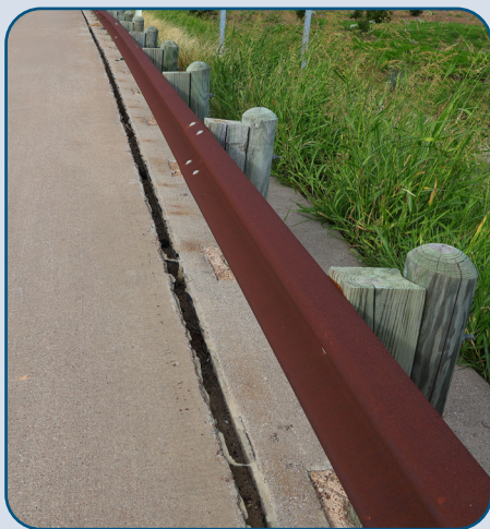
Figure 57: CTP SB Unsealed Longitudinal Joint North of Old Grandbury Rd.
