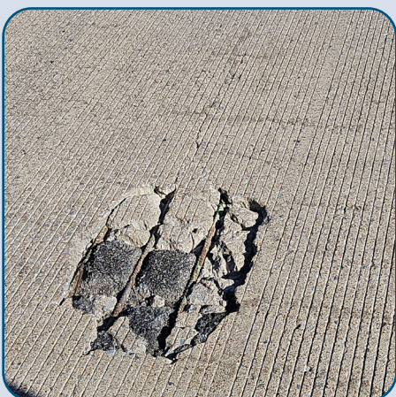
Figure 28: PGBT Deck Deterioration on Bridge Over Lake Ray Hubbard.
