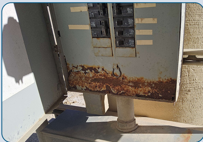
Figure 36: PGBT Brand Road Winter Weather Operation Facility Corrosion.
