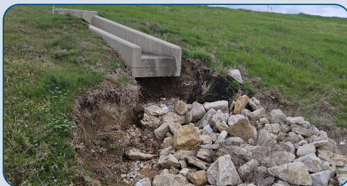
Figure 97: 360T SB Drainage Structure Undermined at N Holland Rd.
