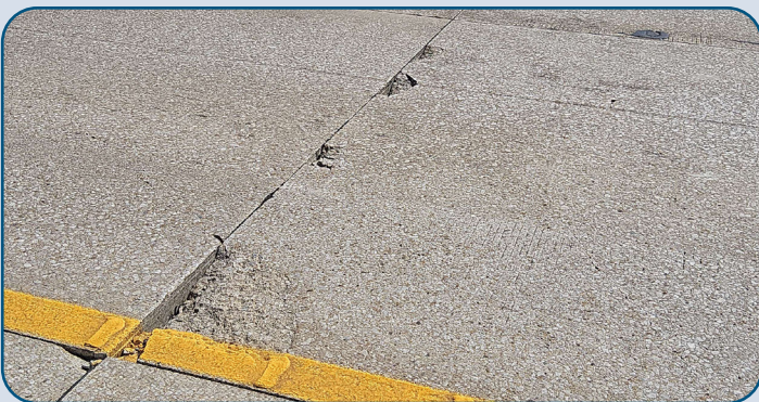
Figure 95: 360T NB Concrete Pavement Cracking and Spalling North of Doryn Dr.
