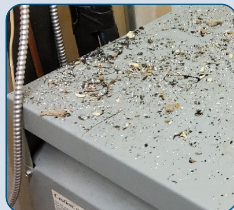
Figure 120: Gleneagles 5910 Insect Infestation.
