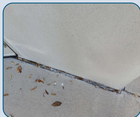
Figure 77: MCLB Fiber Hut Joint Failure.
