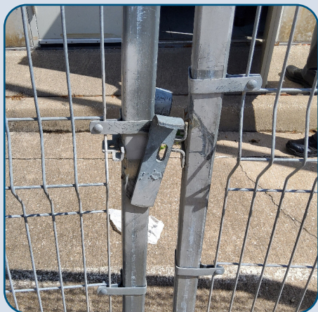
Figure 18: DNT Fiber Hut 1 Uncloseable Gate Lock.
