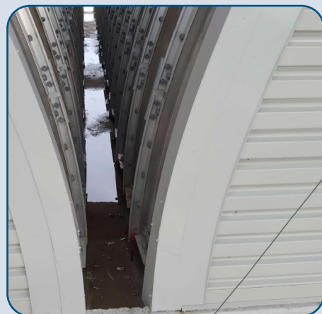
Figure 20: DNT US-380 Winter Weather Operation Facility Roof with Ponding.
