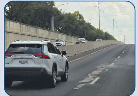
Figure 3: DNT SB Pavement Reflective Cracking and Spalling South of IH 635.
