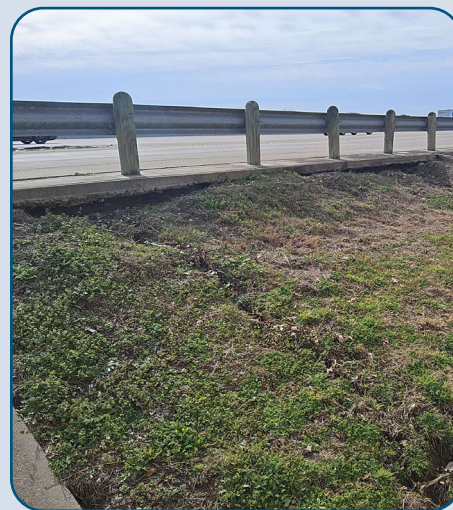
Figure 41: SRT WBML Mow Strip Undermining and Turf Erosion West of Hebron Pkwy.
