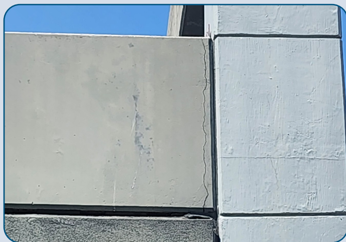
Figure 32: PGBT Midway Road On-Ramp Gantry Panel Crack.
