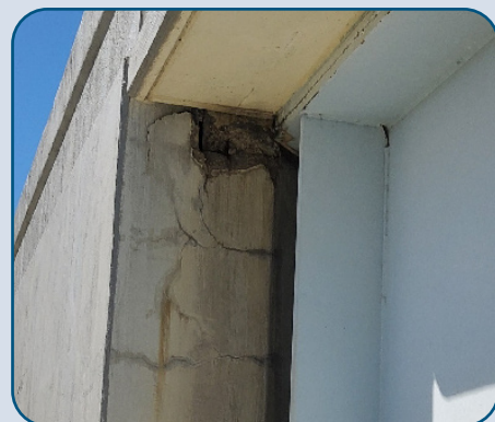
Figure 105: 360T NB Backwall Cracking and Spalling at NE Green Oaks Blvd.
