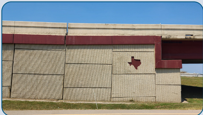
Figure 26: PGBT MSE Wall Racked Panels at IH 635.
