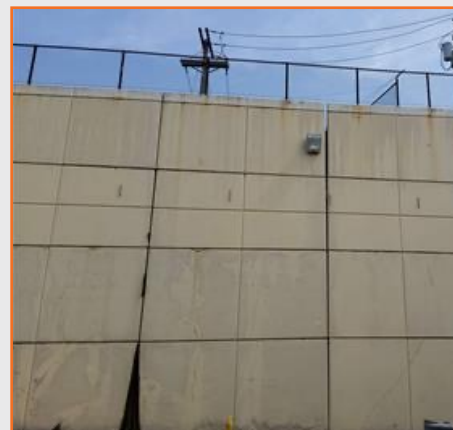
Figure 80: AATT retaining wall panel cracks, spalls and damaged/missing joint seal on west approach to tunnel.
