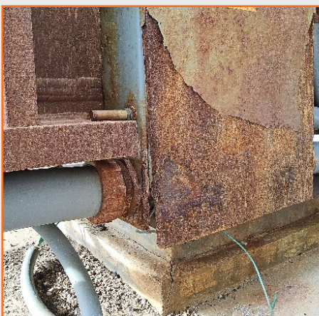
Figure 72: LLTB corroded electrical box.
