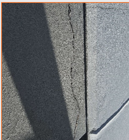
Figure 33: PGBT Midway Road On-Ramp Gantry panel crack.
