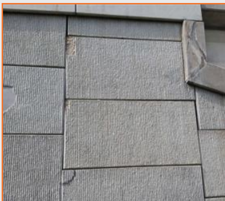
Figure 42: SRT retaining wall spalling NBML at W. Spring Creek Pkwy.
