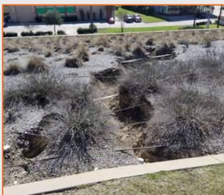
Figure 38: SRT landscape bed erosion NBML at Custer Rd.
