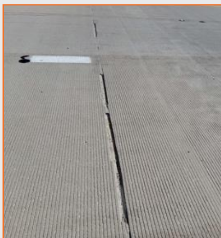
Figure 92: 360T spalling deck at Walnut Creek.
