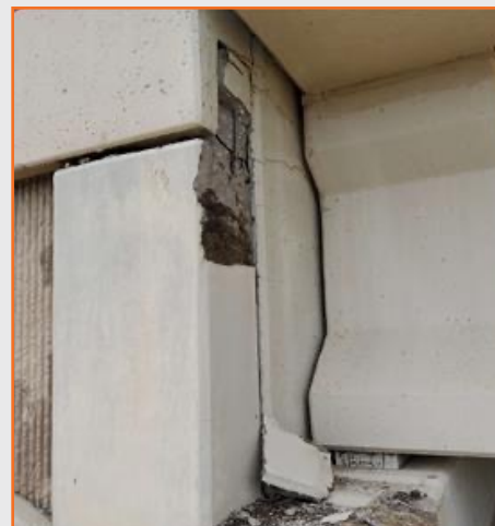
Figure 28: PGBT abutment spalling north of Sandy Lake Rd.
