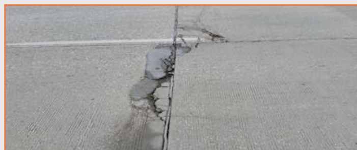
Figure 54: CTP concrete pavement distress at on-ramp from McPherson Blvd.
