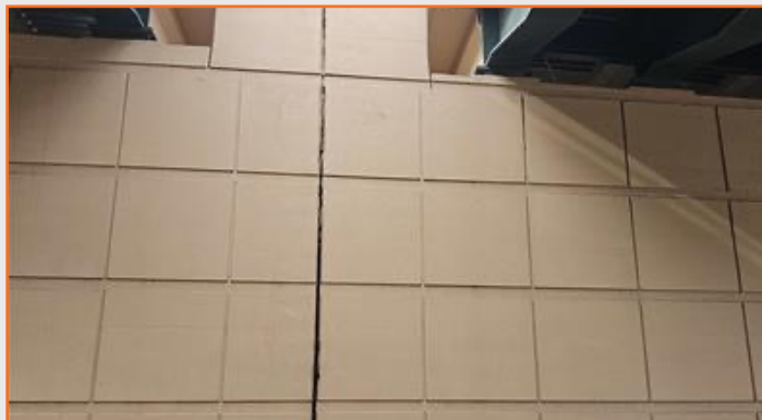
Figure 56: CTP retaining wall panels unsealed NBML at Old University Dr.
