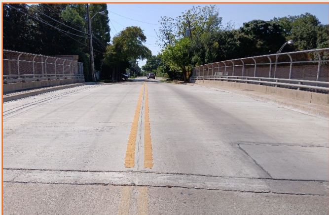
Figure 109: Dallas North Tollway at Park Lane – Partial Depth Deck Replacement.
