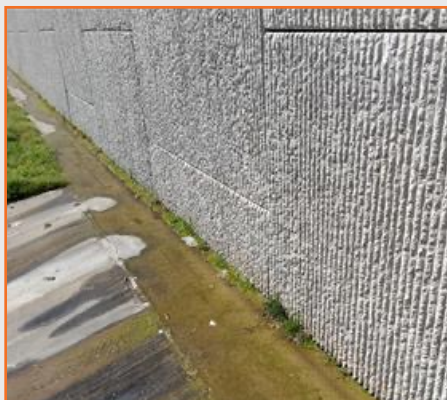
Figure 43: SRT retaining wall with considerable water seepage NBML at Custer Rd.
