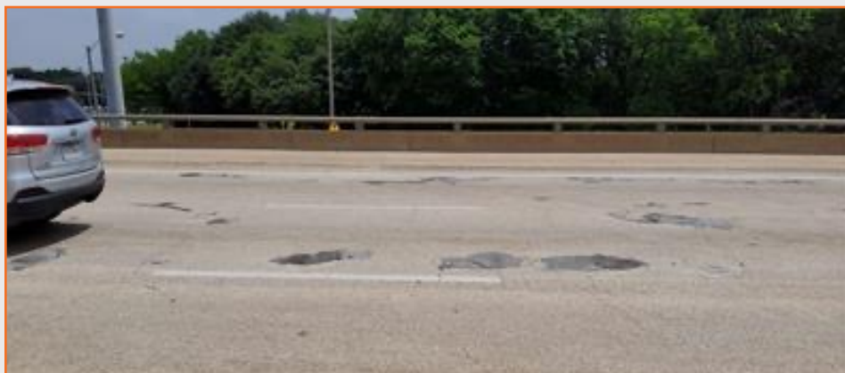
Figure 9: DNT bridge deck deterioration at Lomo Alto Dr.
