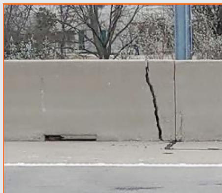
Figure 36: SRT concrete rail cracking NBML south of Medical Center Dr.
