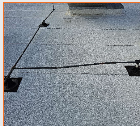
Figure 106: Gleneagles 5900 Plano Parkway damaged RTU condensate drain pipe.
