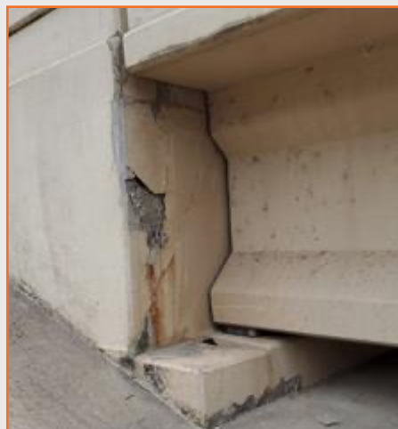
Figure 46: SRT abutment backwall spalling at W. Rowlett Creek.
