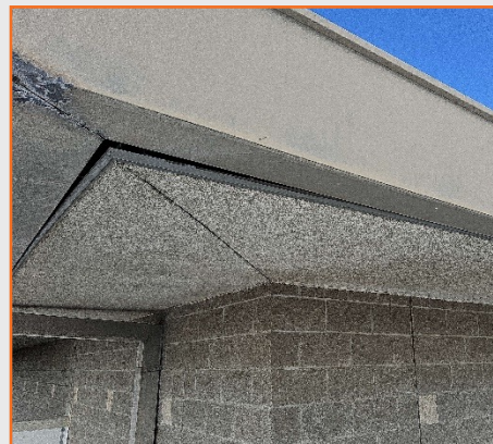
Figure 108: Gleneagles 5910 Plano Parkway sagging/separated soffit.
