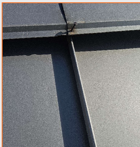
Figure 100: Plano Operations Center loose roof fastener.
