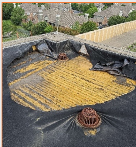
Figure 32: PGBT Renner Road On-Ramp Gantry roof deterioration.
