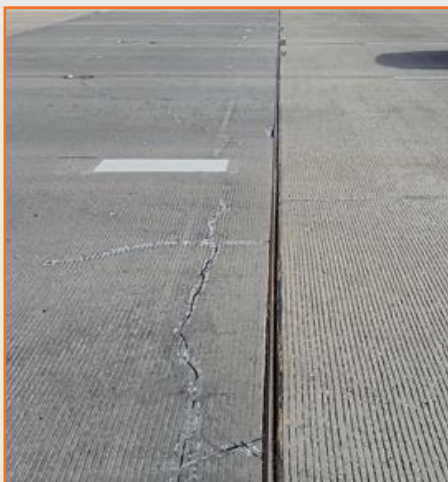
Figure 45: SRT closed bridge joint with cracked approach slab pavement at Paige/Plano Pkwy.
