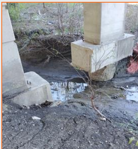
Figure 26: PGBT bridge erosion at Rowlett Creek.
