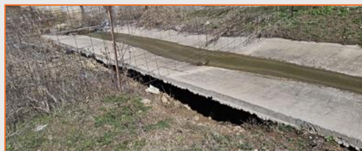
Figure 53: CTP drainage flume undermining SBML north of FM 1187.
