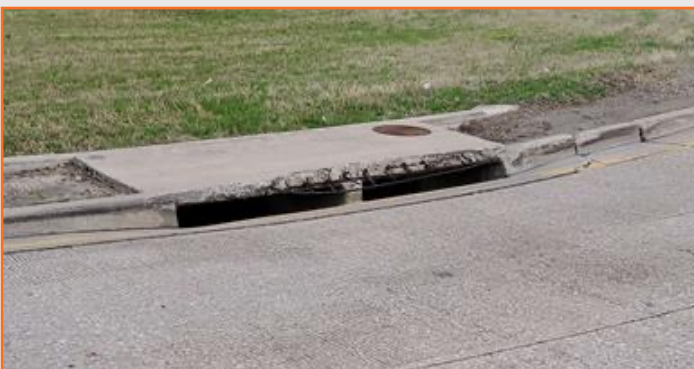
Figure 90: 360T concrete curb inlet damage at Kingswood Blvd. SB U-Turn.
