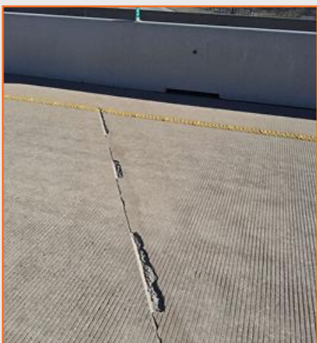
Figure 57: CTP approach slab construction joint spalling at FM 1902.
