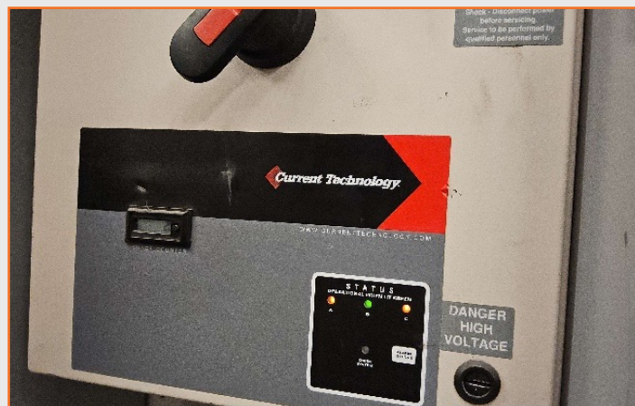
Figure 84: AATT Main Electrical Room failed surge protection device.
