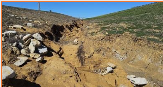
Figure 88: 360T ditch line erosion at Heritage Pkwy.
