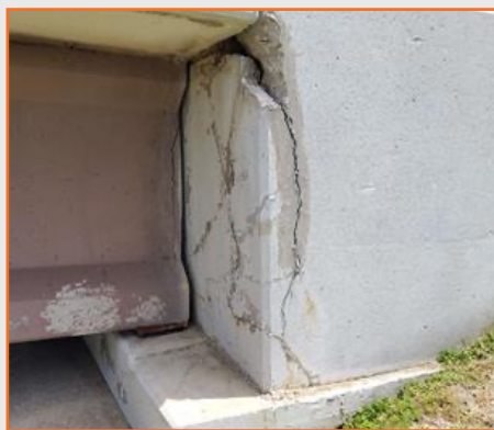
Figure 10: DNT abutment backwall cracking at IH-635.
