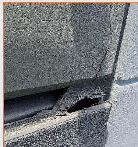
Figure 34: PGBT Midway Road On-Ramp Gantry panel separation.
