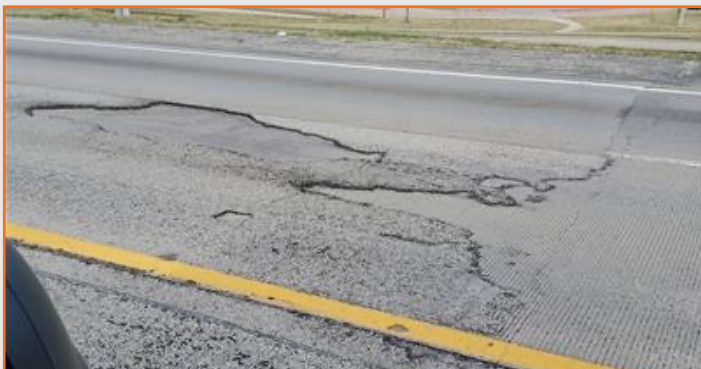
Figure 87: 360T asphalt overlay pavement deterioration NBML south of SE Green Oaks Blvd./Kingwood Blvd.
