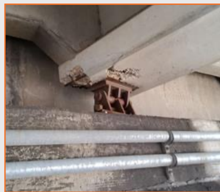
Figure 11: DNT concrete beam end damage with exposed reinforcement at Forest Ln.
