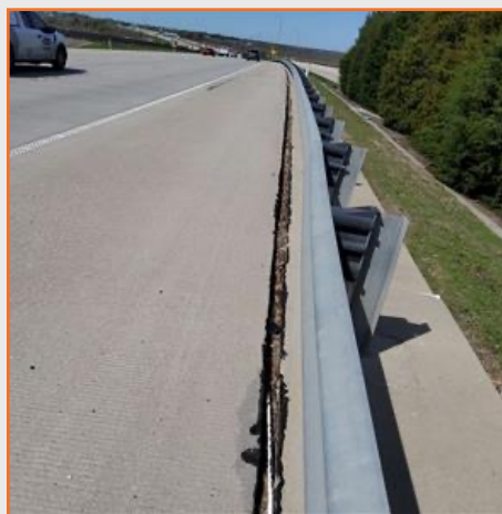
Figure 21: PGBT pavement and mow strip separation NBML at Merritt Rd.
