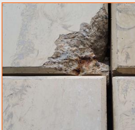
Figure 79: AATT retaining wall panel spall on east approach to tunnel.
