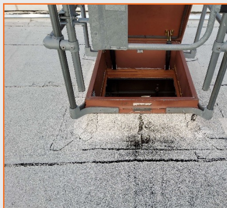
Figure 105: Gleneagles 5900 Plano Parkway loose roof access handrail.
