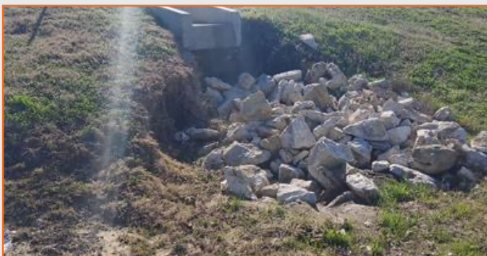
Figure 89: 360T drainage culvert outfall erosion at N. Holland Rd.
