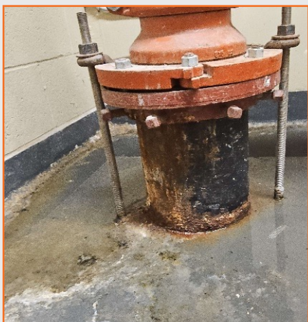
Figure 99: Plano Operations Center corroded fire riser pipe.
