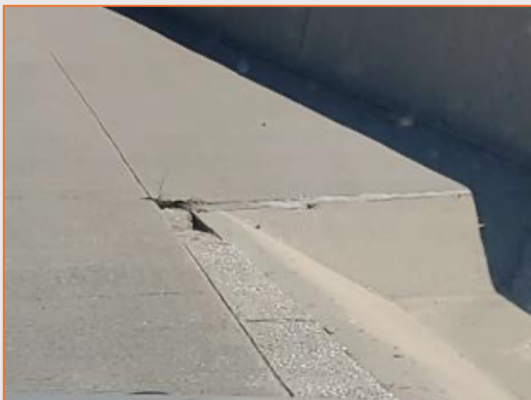
Figure 67: LLTB concrete flume spalling EBML on east approach to bridge.
