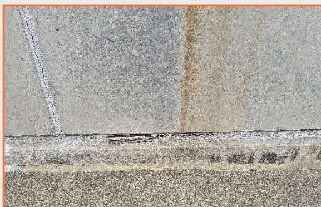
Figure 48: SRT MLG1 failed joint sealant.
