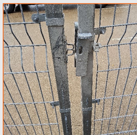
Figure 17: DNT MLP2 Fiber Hut inoperable gate lock.
