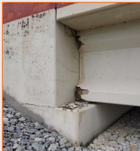
Figure 27: PGBT concrete beam spalling near future Valwood Pkwy.
