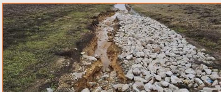
Figure 51: CTP ditch erosion SBML embankment erosion NBML north of W. FM 917.
