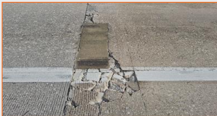
Figure 86: 360T concrete pavement deterioration SBFR north of E. Sublett Rd./W. Camp Wisdom Rd.
