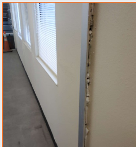
Figure 30: PGBT MLP9 wall separation/shifting.
