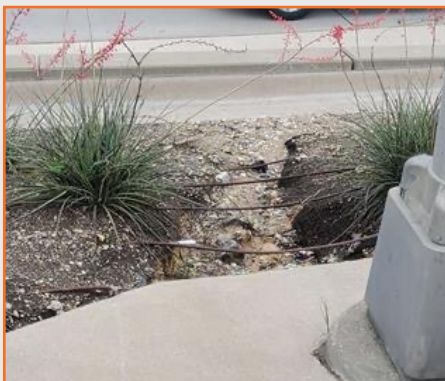
Figure 5: DNT erosion NBML south of Eldorado Pkwy.
