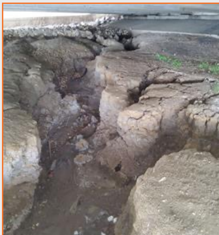
Figure 69: LLTB east abutment erosion.
