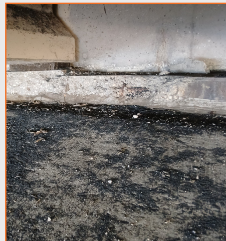
Figure 71: LLTB east abutment spalling with exposed reinforcement.
