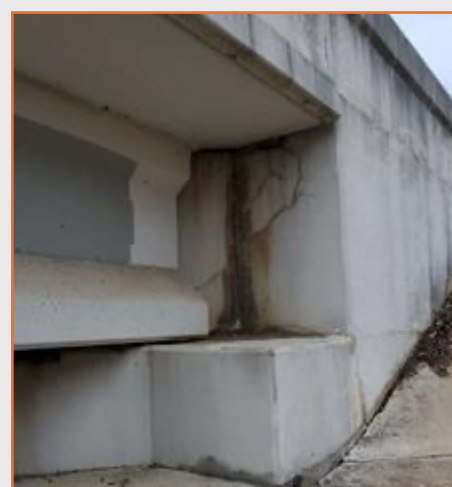
Figure 94: 360T abutment backwall cracking at Fish Creek.
