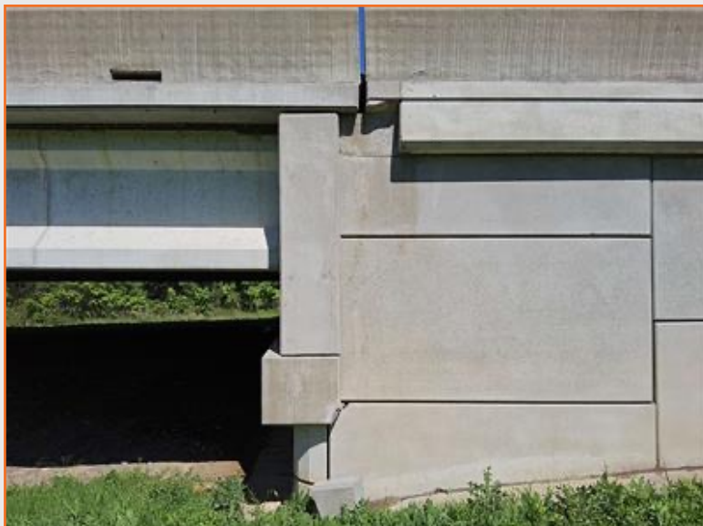
Figure 68: LLTB retaining wall coping damage.
