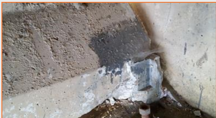
Figure 66: MCLB west abutment concrete beam spalling.
