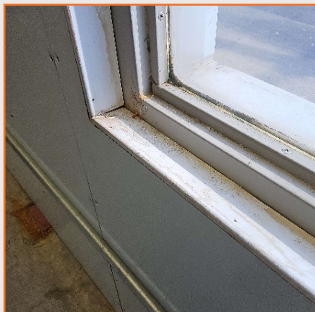
Figure 12: DNT MLG1 water infiltration.
