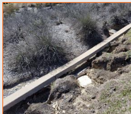
Figure 37: SRT turf and landscape bed erosion NBML at near Custer Rd.
