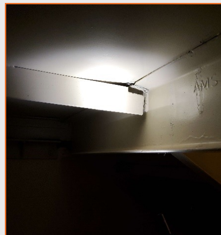
Figure 31: PGBT MLP9 stair frame separation/settling.
