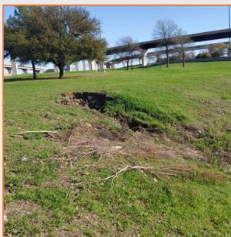
Figure 18: PGBT erosion SBML at IH-30 in Garland, TX.
