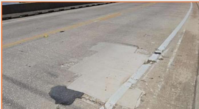
Figure 65: MCLB east abutment approach slab surface spalling.
