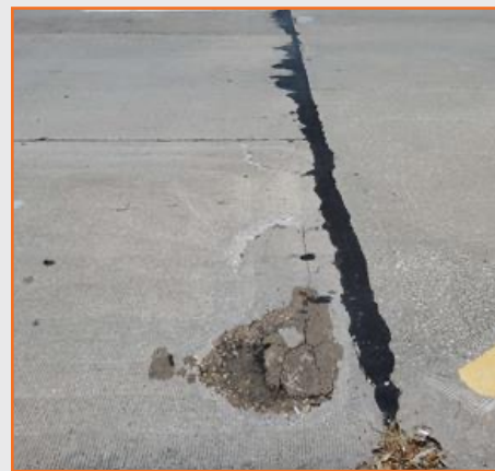
Figure 76: AATT concrete pavement distress.
