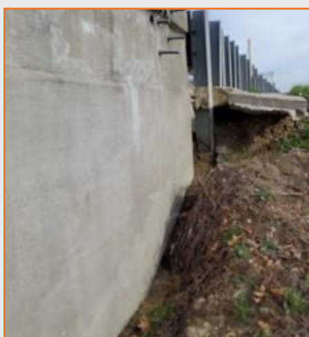
Figure 93: 360T erosion adjacent to approach slab guardrail at Bowman Branch.
