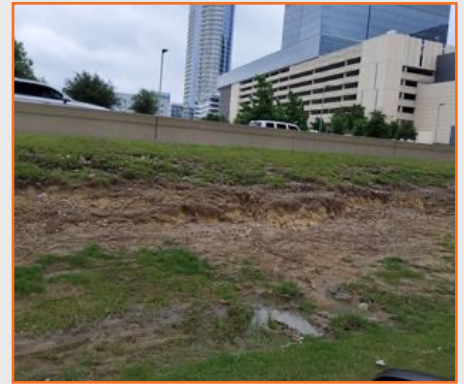
Figure 4: DNT turf erosion SBML south of SRT.
