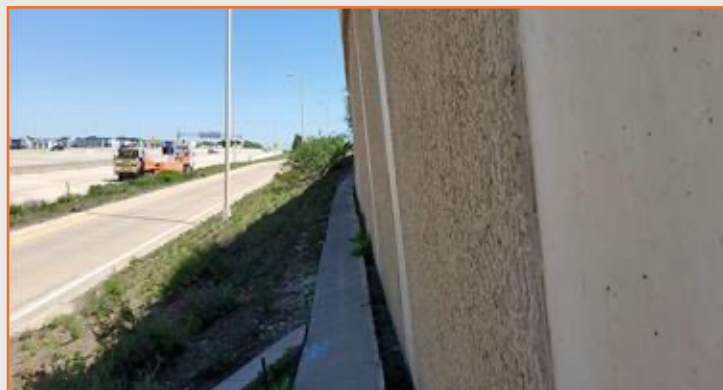
Figure 25: PGBT soundwall movement adjacent to NB exit ramp to Frankford Rd.
