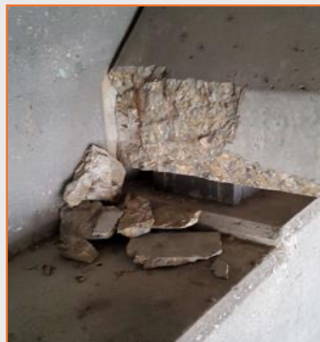
Figure 47: SRT bridge beam spalling with exposed reinforcement at W. Rowlett Creek.
