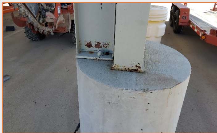
Figure 103: Plano Operations Center outbuilding rust.
