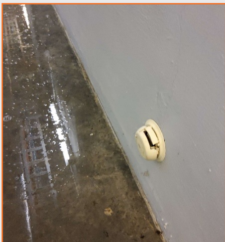
Figure 29: PGBT MLP7 tunnel damaged CO sensor.
