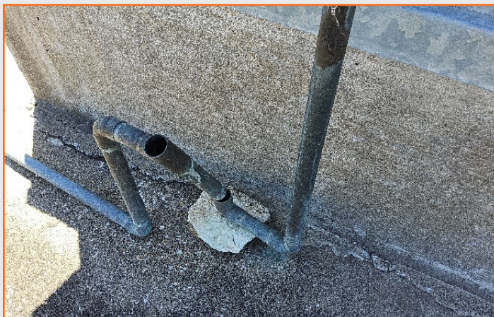
Figure 81: AATT broken RTU condensate drain pipe.
