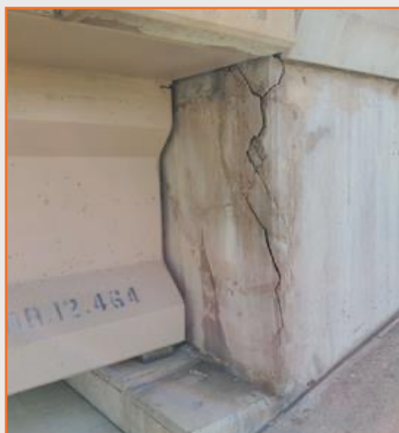
Figure 58: CTP abutment backwall cracking at IH-20.
