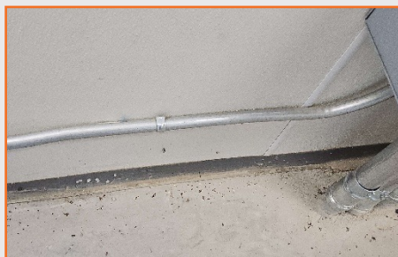
Figure 49: SRT MLG3 insect infestation.
