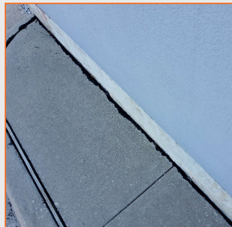
Figure 13: DNT MLP3 joint sealant failure.
