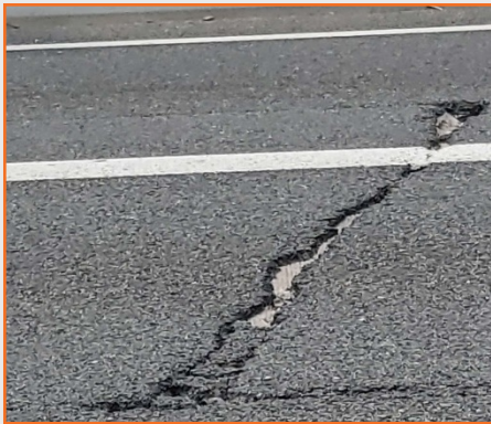
Figure 2: DNT pavement cracking and spalling SBML north of IH-635.
