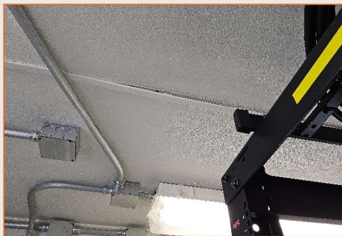
Figure 63: CTP MLG1 peeling ceiling seam strip.
