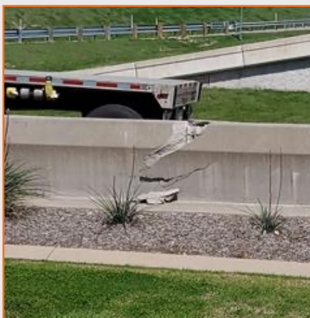
Figure 22: PGBT concrete rail damage WBML at Lavon Dr.
