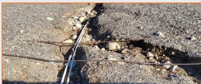
Figure 52: CTP landscape erosion NBML at IH 20.
