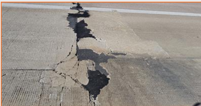
Figure 85: 360T concrete pavement deterioration NBML north of Lone Star Rd.
