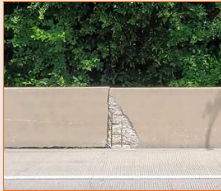
Figure 3: DNT concrete rail damage NBML south of Maple Ave.
