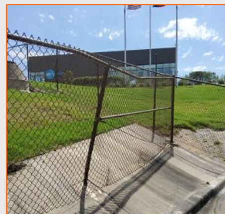
Figure 78: AATT access control fence damage.
