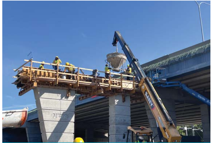
Pouring concrete for bridge cap
