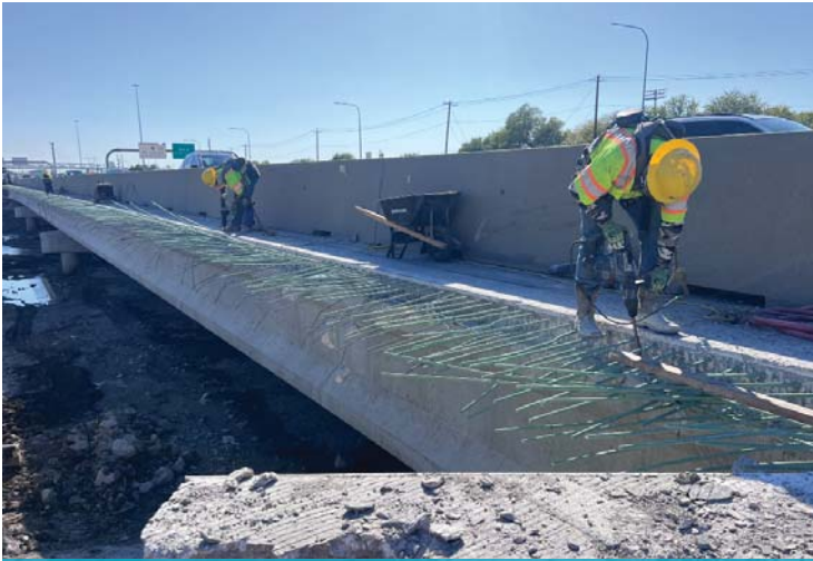
Hand chipping for bridge widening
