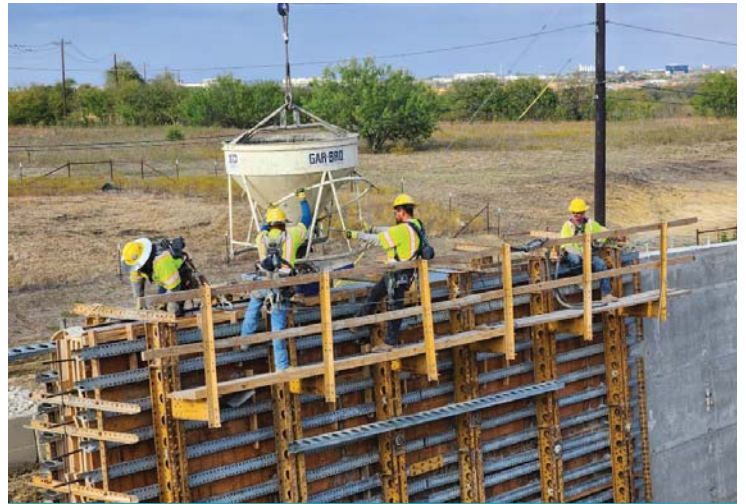
Concrete placement
