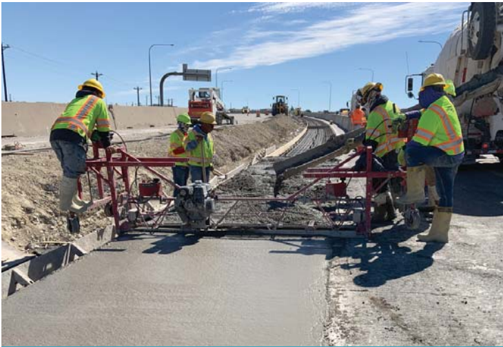
Concrete placement
