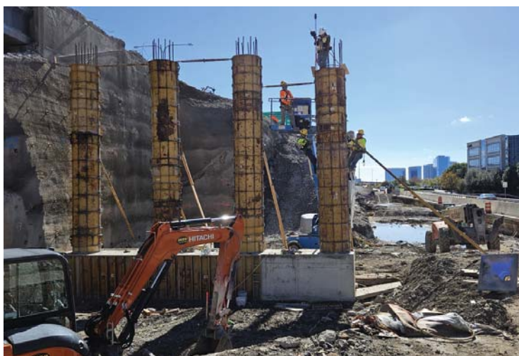
Forming bridge columns
