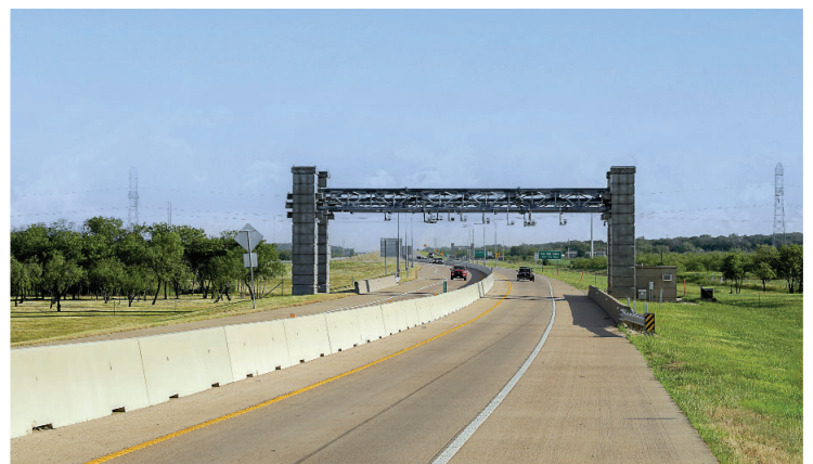
Existing toll gantry
