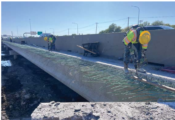
Hand chipping for bridge widening
