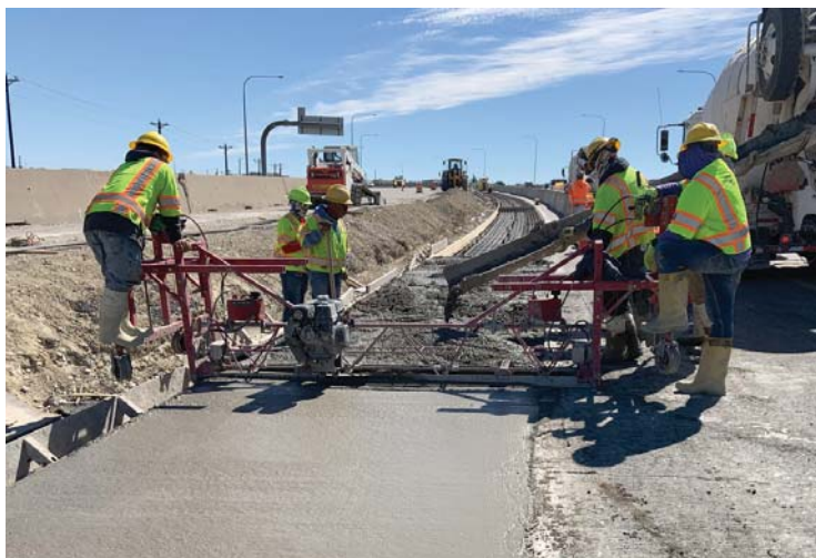
Concrete placement
