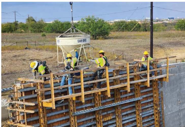
Concrete placement
