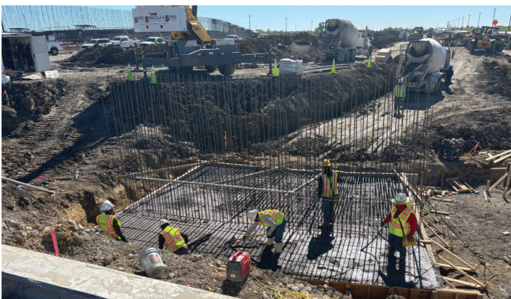
Pouring concrete for future wall foundations
