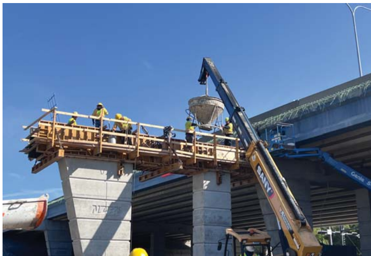
Pouring concrete for bridge cap
