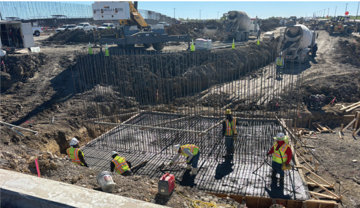
Pouring concrete for future wall foundations
