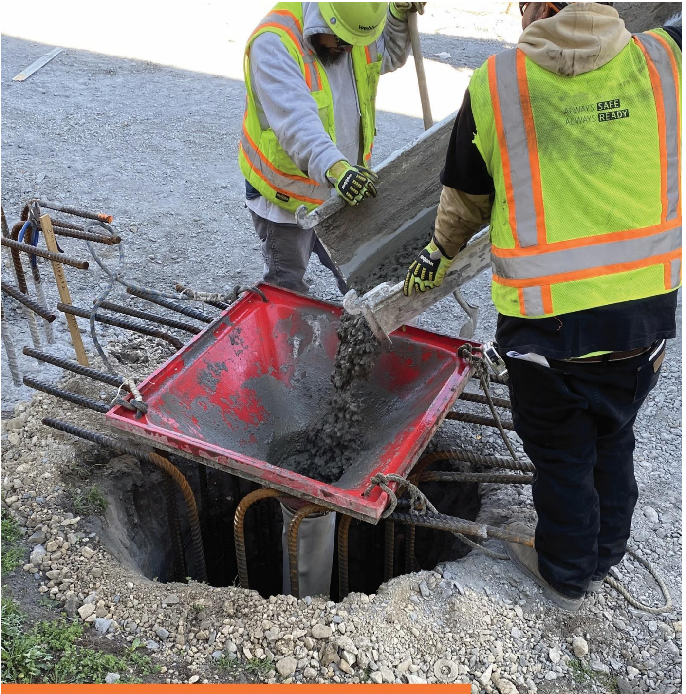
Placing concrete for drilled shaft foundation
