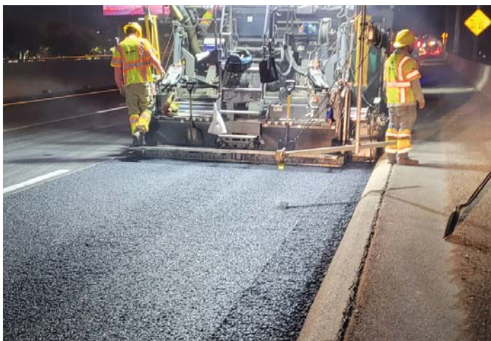
Placing new driving surface on northbound DNT
