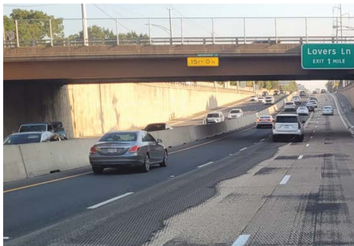
Completed left lane with new driving surface
