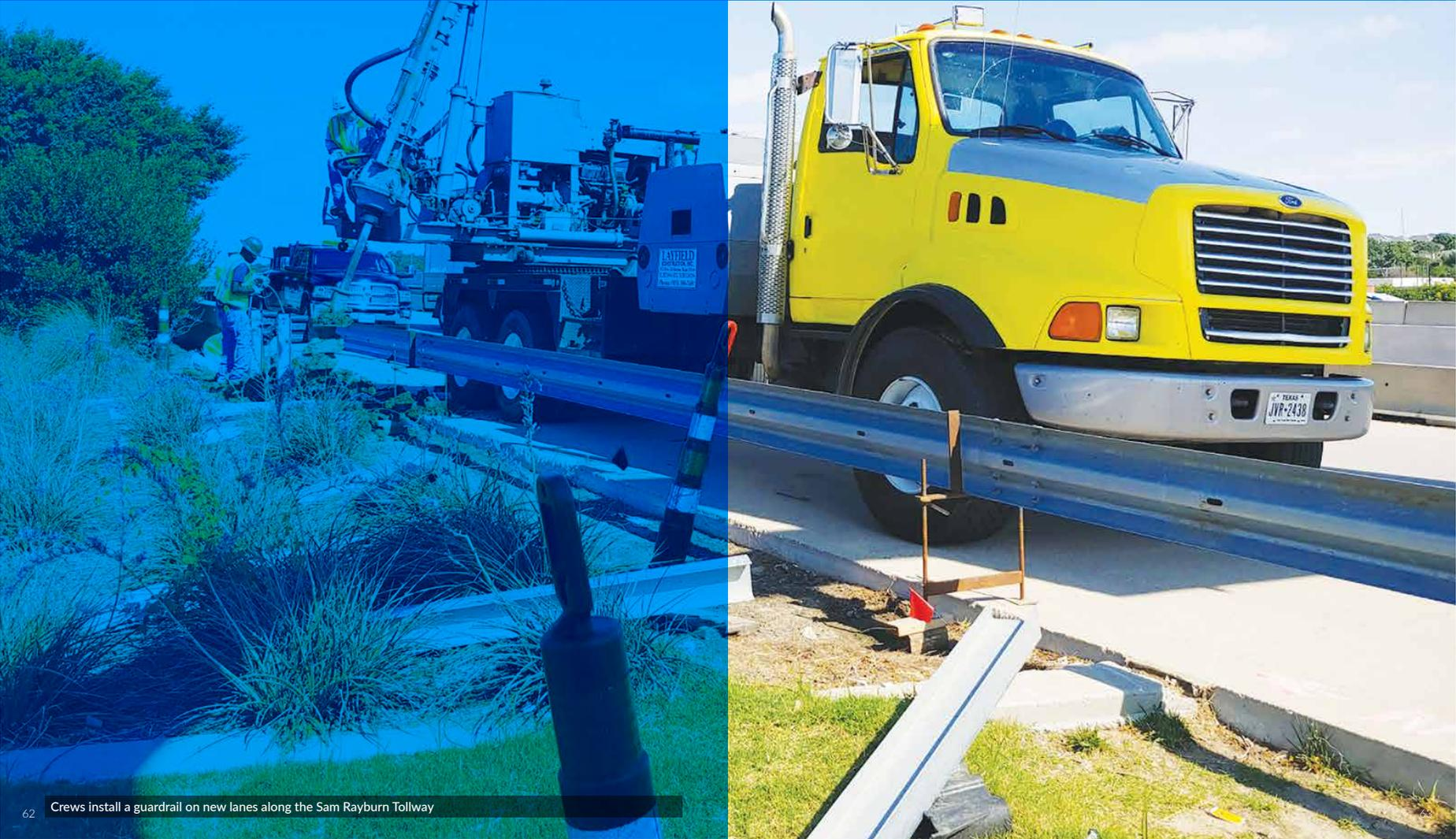
62 Crews install a guardrail on new lanes along the Sam Rayburn Tollway
