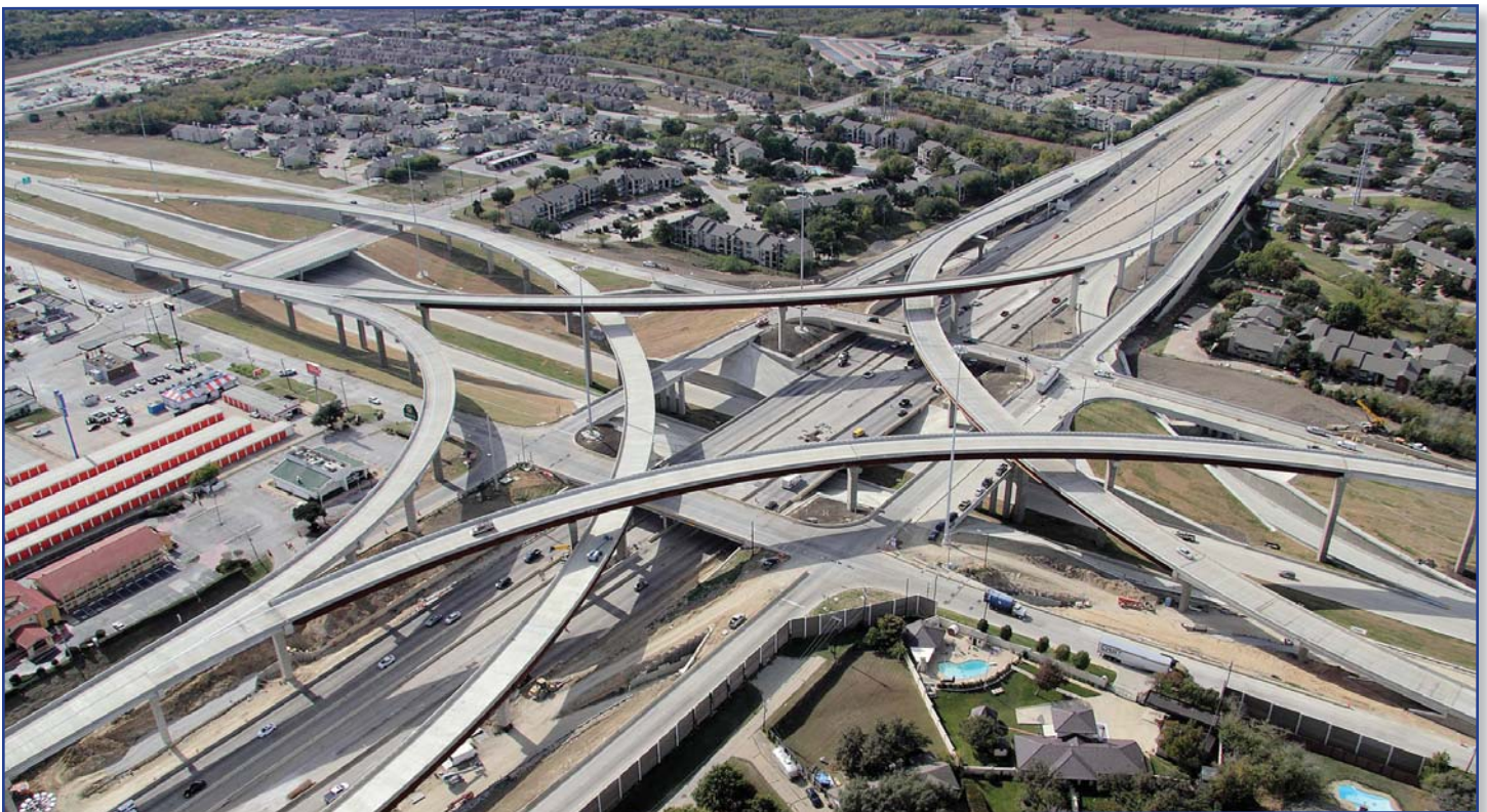
Looking north at Western Extension/I-30 interchange.
