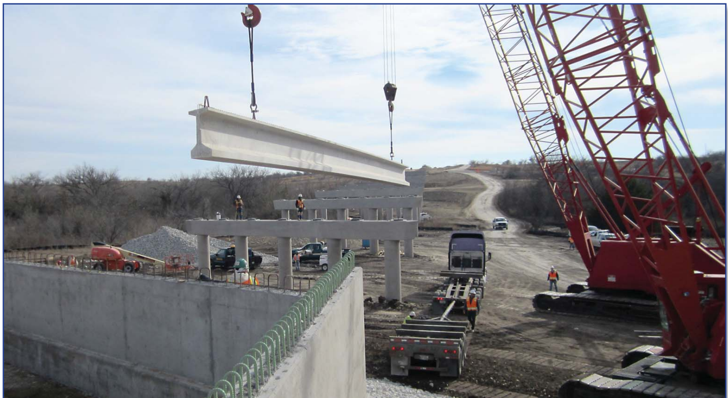
Crews place bridge beams at County Road 1015 in Johnson County.
