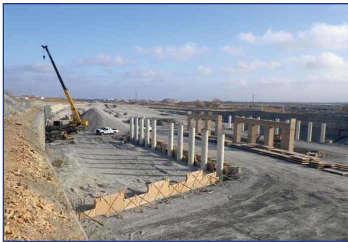
CTP retaining wall construction near Oakmont Boulevard in Fort Worth.
