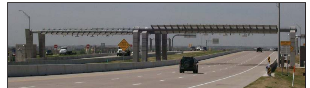
Sam Rayburn Tollway Main Lane Toll Gantry
