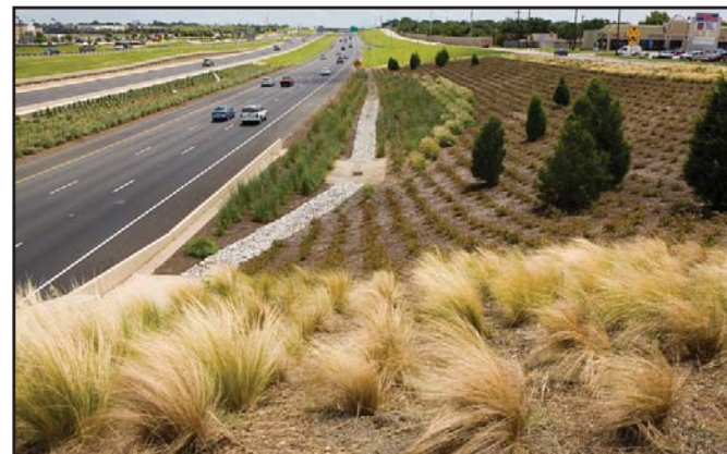
President George Bush Turnpike Interchange at Josey Lane
