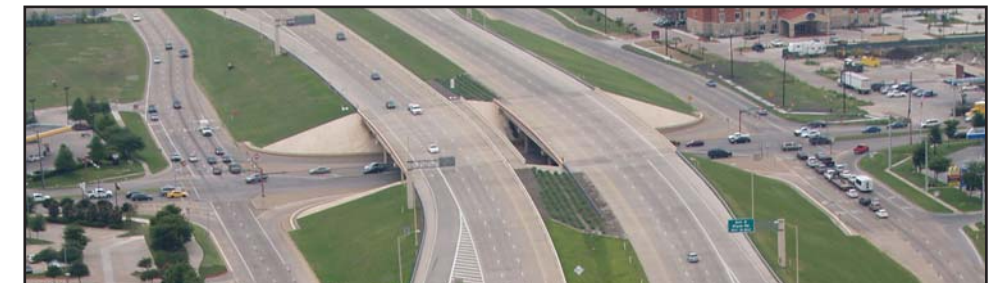
President George Bush Turnpike at Coit Road Overpass
