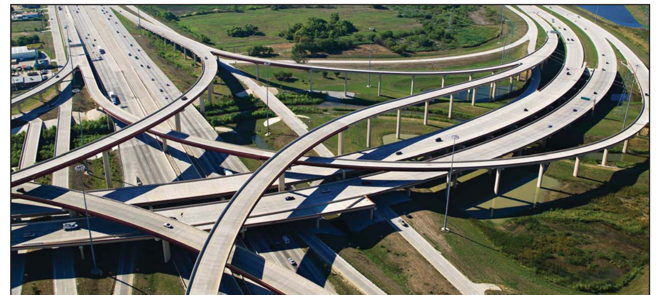
President George Bush Turnpike and Highway 35E Interchange
