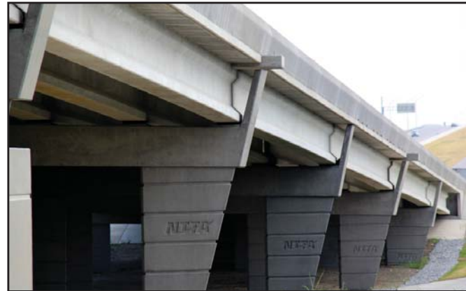
Sam Rayburn Tollway at Exchange Parkway
