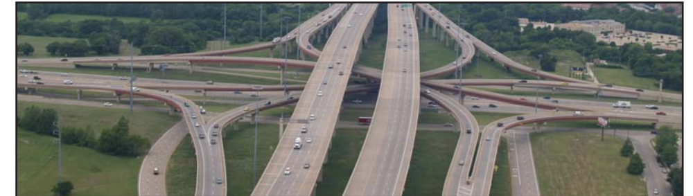
Dallas North Tollway and President George Bush Turnpike Interchange
