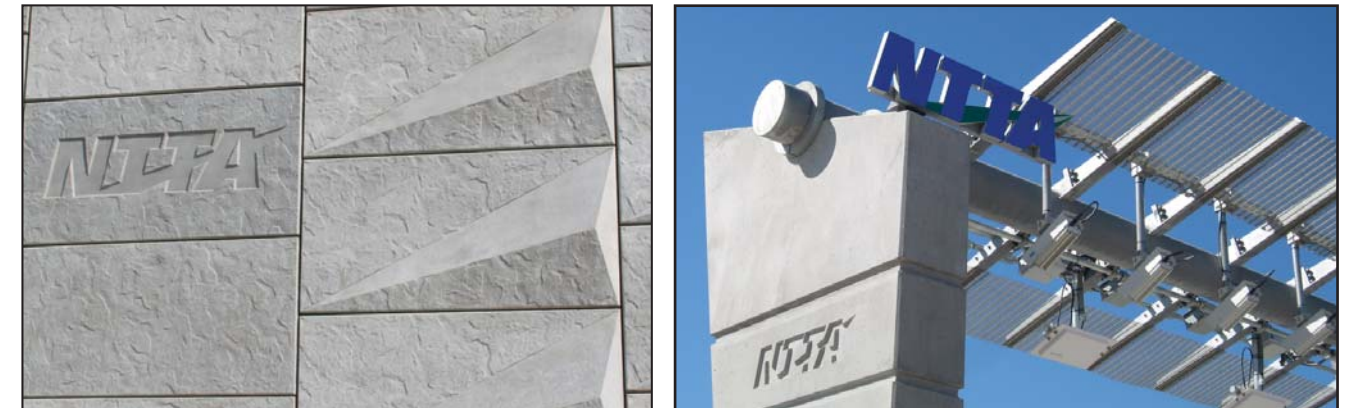
MSE Wall on Sam Rayburn Tollway
