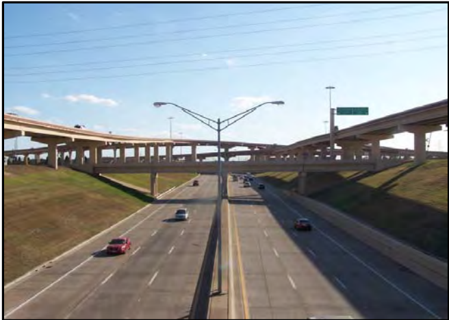
Photo 1. Looking south along DNT at PBGT interchange (project begin).
