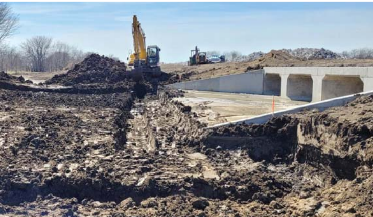
Excavating culvert crossing at the DNT 4B frontage road
