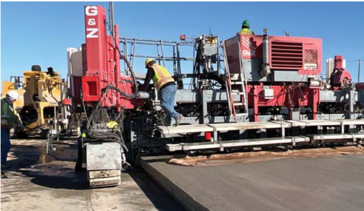
Placing pavement at the DNT extension over US 380
