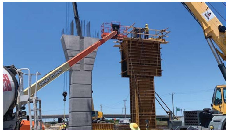
Pouring a column for the northbound main lanes.
