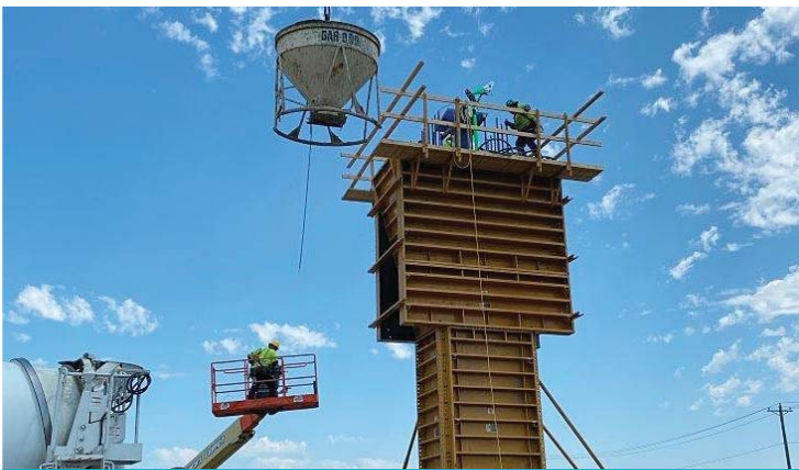
Pouring columns on the south end of the project.
