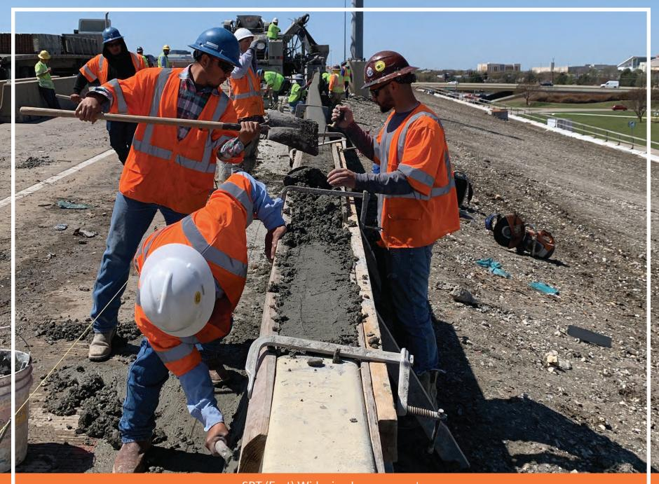
SRT (East) Widening Improvement Placing concrete for traffic rail
