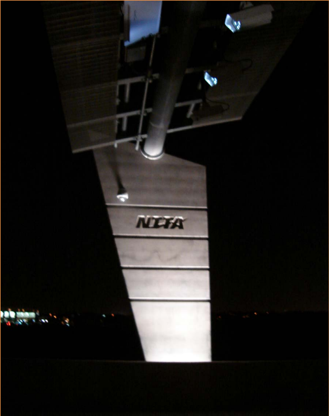
NTTA Gantry at Night
