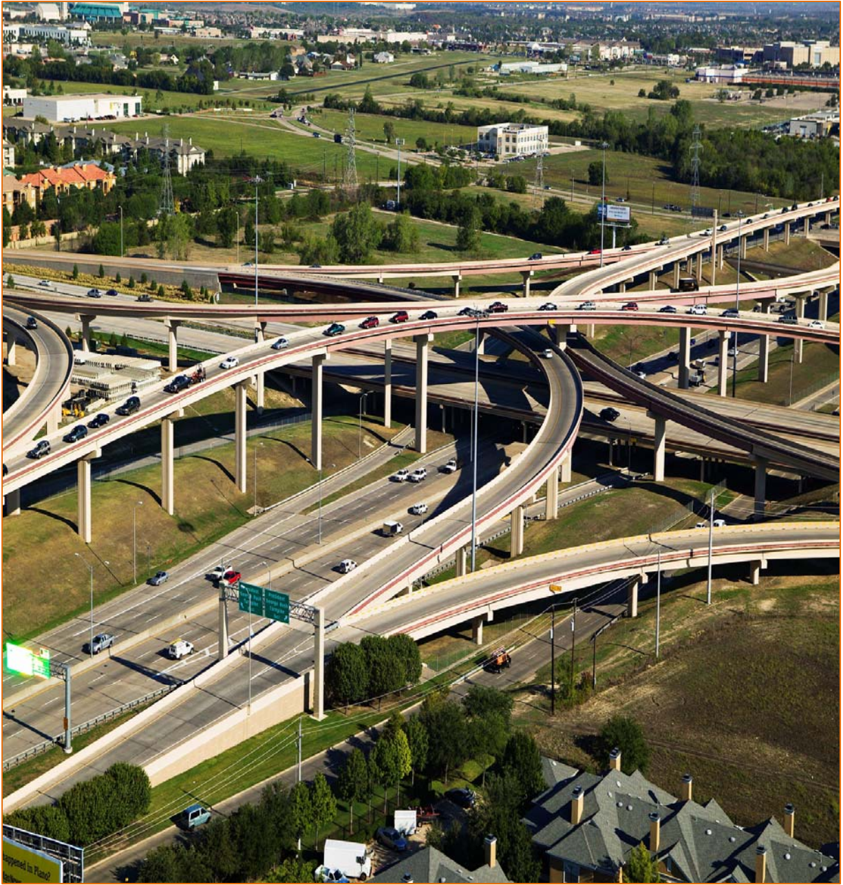
Dallas North Tollway North going under President George Bush Turnpike Interchange
