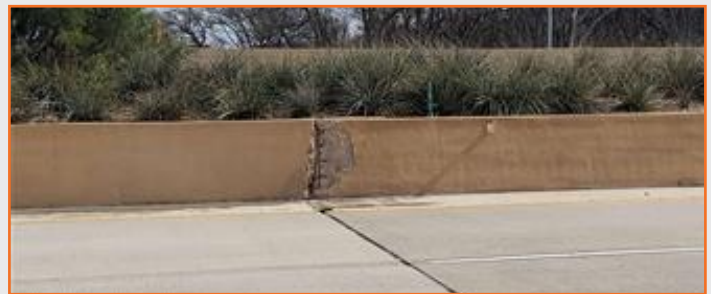
Figure 50: CTP concrete barrier SBML south of Arborlawn Dr.
