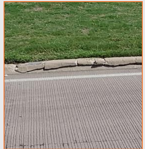
Figure 40: SRT curb damage SBFR south of W. Exchange Pkwy.
