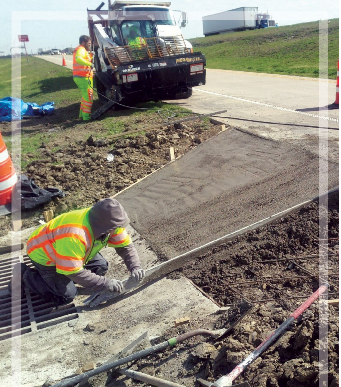
Pouring concrete for inlet drain
