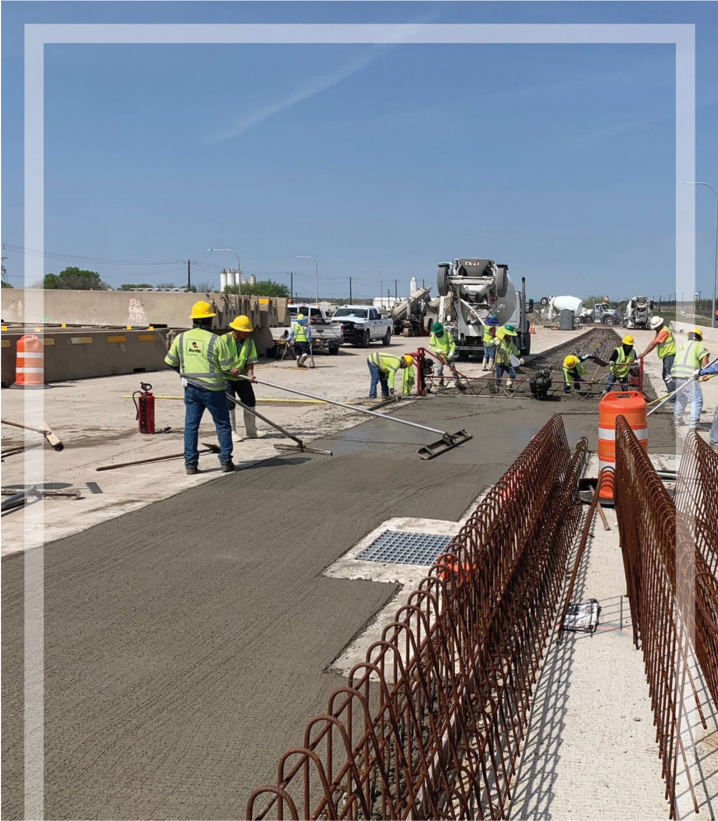
Placing concrete on Dallas North Tollway extension bridge over US 380
