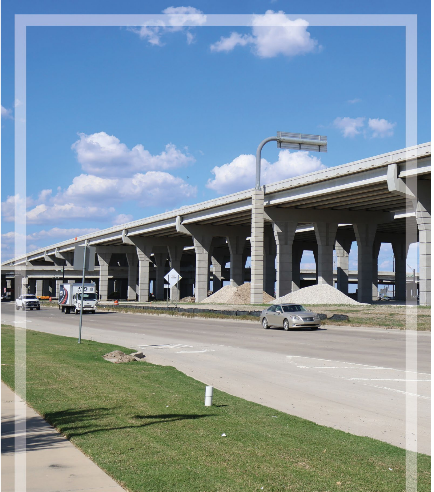
Dallas North Tollway extension bridge over US 380
