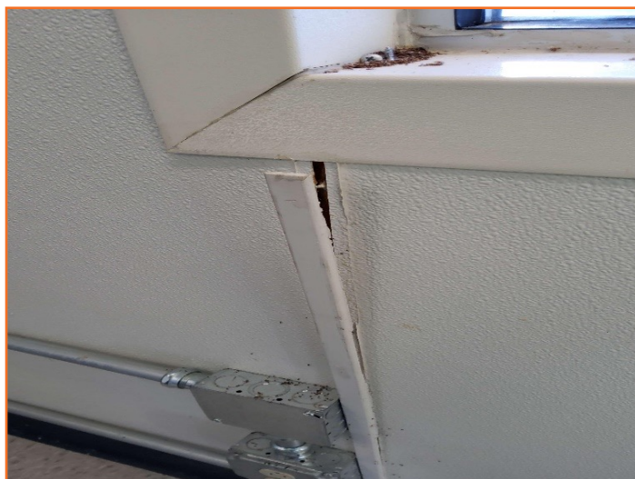
Figure 38: CTP MLG 1 – wall trim peeling away
