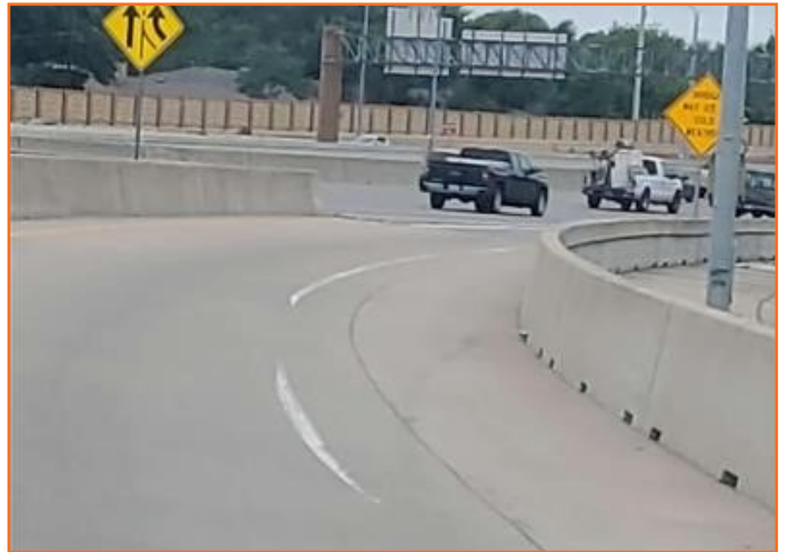
Figure 7: DNT faded pavement markings NBML N. of IH-635
